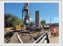
the successful installation of eight temporarily cased CIDH piles. The project anticipated having wet piles, but only encountered one wet pile which was poured without any anomalies. The other piles were constructed without issues.
