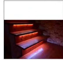
(F) UNDER STEP 4" HAND RAILS STRIP LIGHTS TO ILLUMINATE STEPS (T.B.D. BY ARCH)
