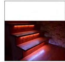
(F) UNDER STEP & HAND RAILS STRIP LIGHTS TO ILLUMINATE STEPS (T.S.D. BY ARCH)
