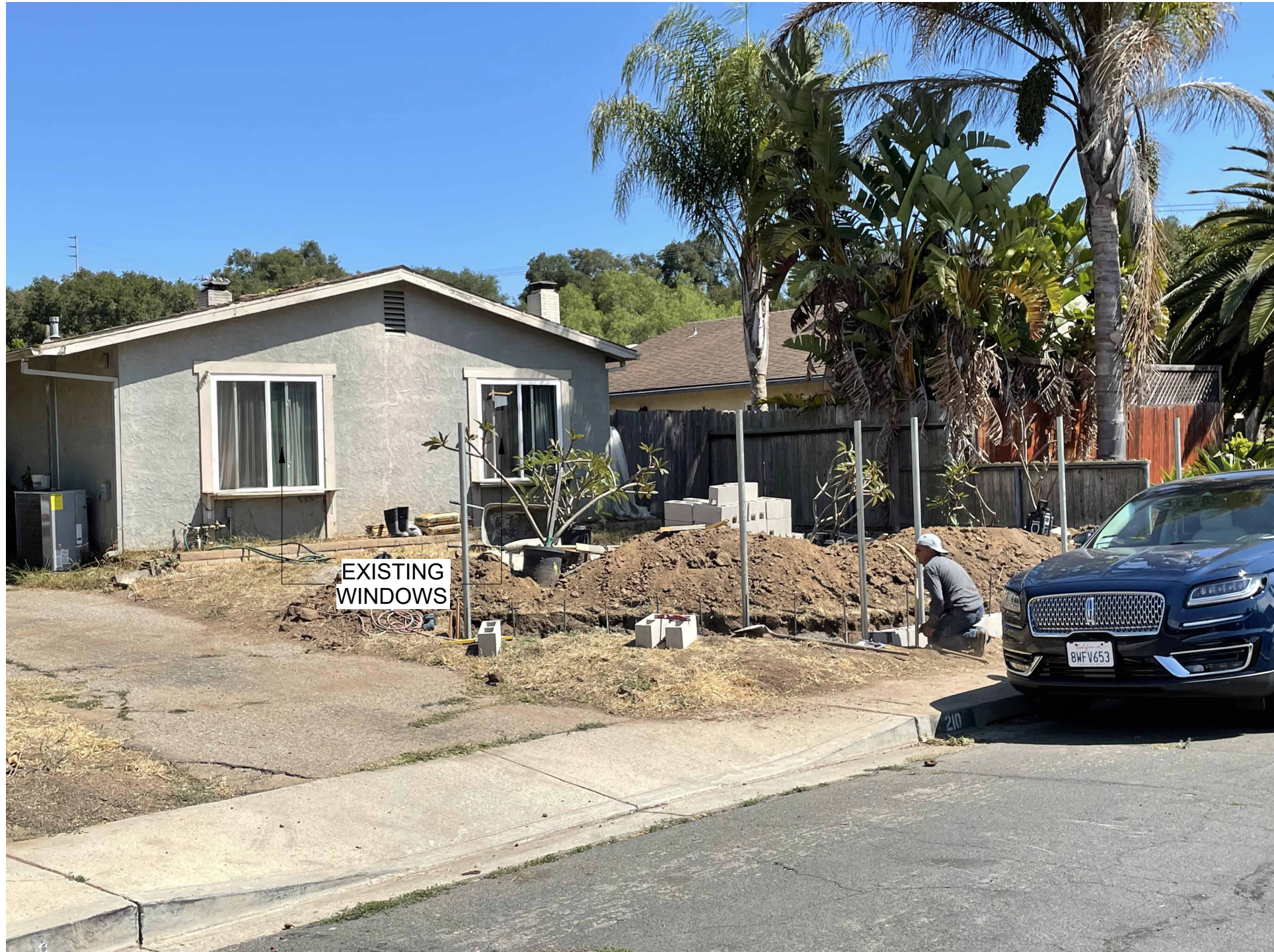
FENCE IN CONSTRUCTION
