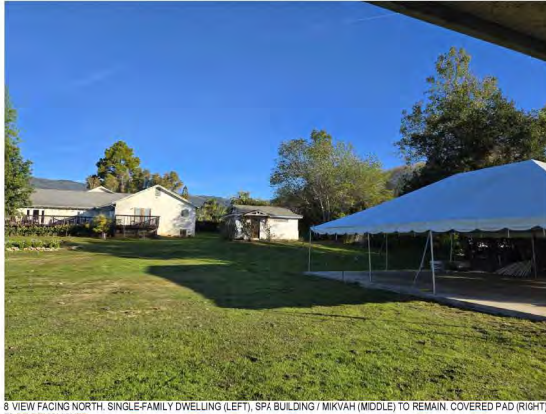
8. VIEW FACING NORTH. SINGLE-FAMILY DWELLING (LEFT), SPA BUILDING / MIKVAH (MIDDLE) TO REMAIN. COVERED PAD (RIGHT) TO BE DEMOLISHED
