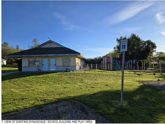
7. VIEW OF EXISTING SYNAGOGUE / SCHOOL BUILDING AND PLAY AREA
