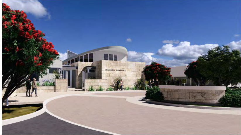
VIEW OF THE WEST FACADE FROM DRIVEWAY ENTRY INTO NEW DROP-OFF ROUNDABOUT
