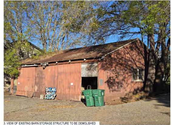
3. VIEW OF EXISTING BARN STORAGE STRUCTURE TO BE DEMOLISHED
