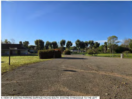
4. VIEW OF EXISTING PARKING SURFACE FACING SOUTH, EXISTING SYNAGOGUE TO THE LEFT
