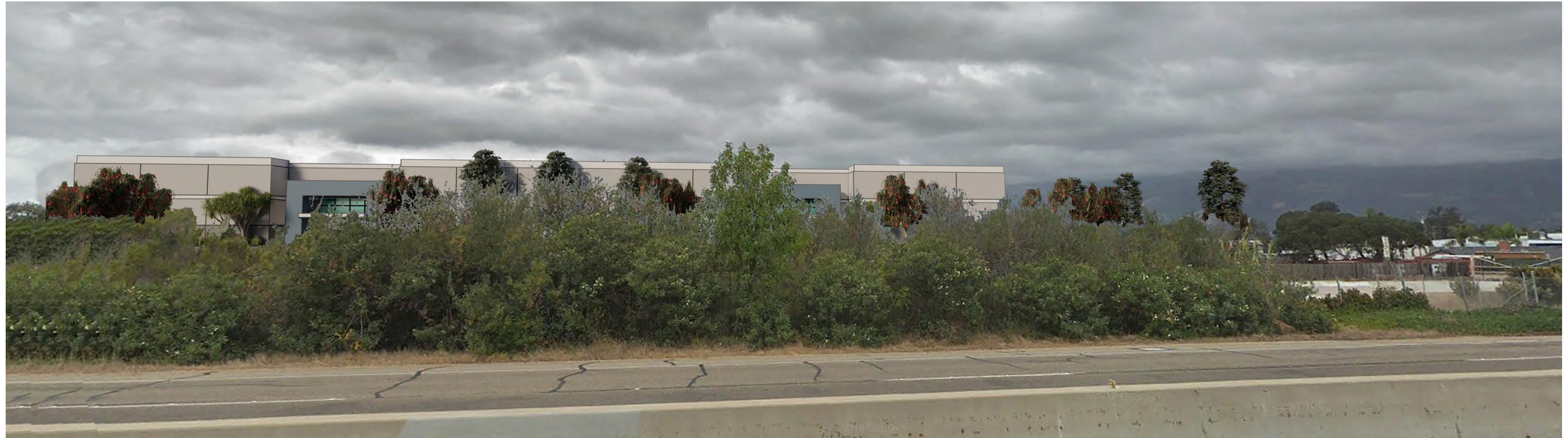
① VIEW FROM HIGHWAY 217 - SITE AND BUILDING ALTERNATE
