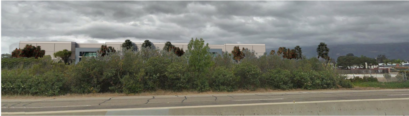
① VIEW FROM HIGHWAY 217 - SITE AND BUILDING ALTERNATE
