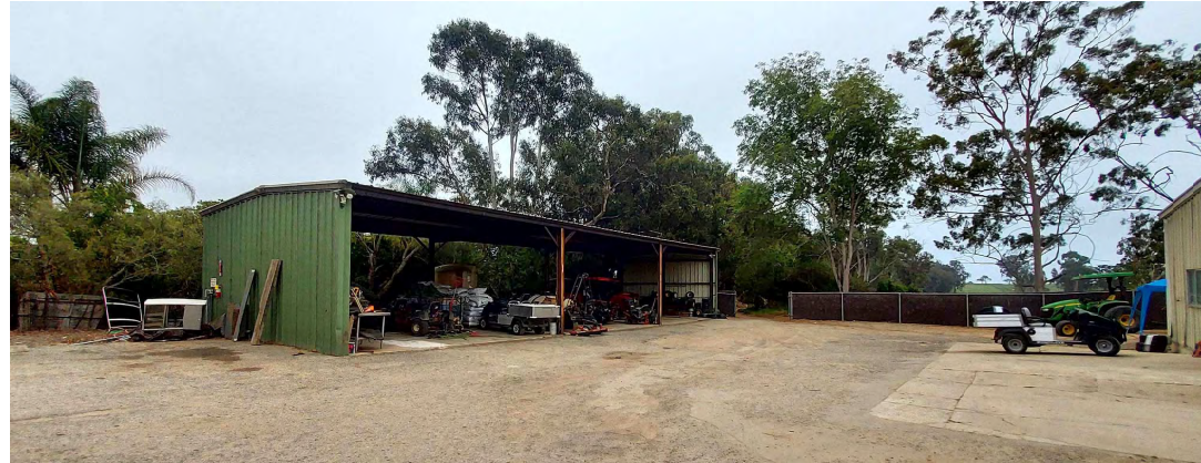
1 LARGE STORAGE SOUTH-EAST VIEW
