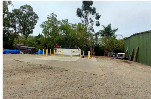
3 FUEL STATION EAST VIEW
