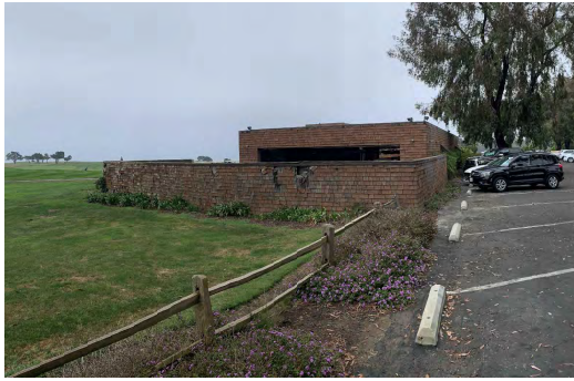
5 CART STORAGE WEST VIEW
