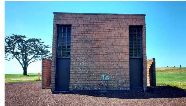
2 COMFORT STATION SOUTH VIEW
