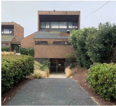
6 CLUB HOUSE BASEMENT NORTH ENTRANCE
