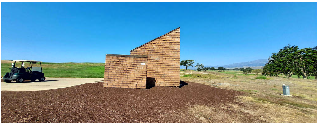
1 COMFORT STATION WEST VIEW (EAST VIEW SIMILAR)
