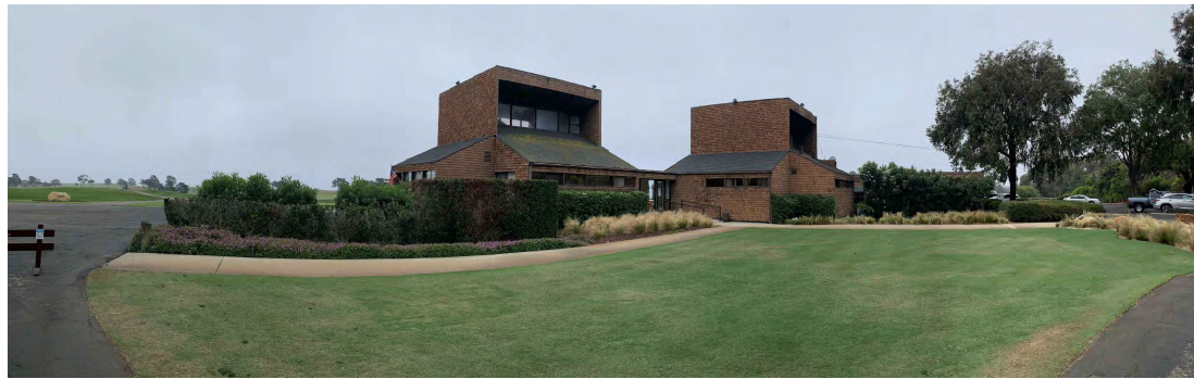
4 CLUB HOUSE WEST VIEW
