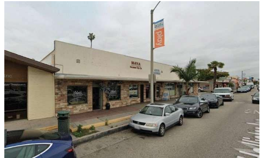
View of property looking East on Hollister Ave
