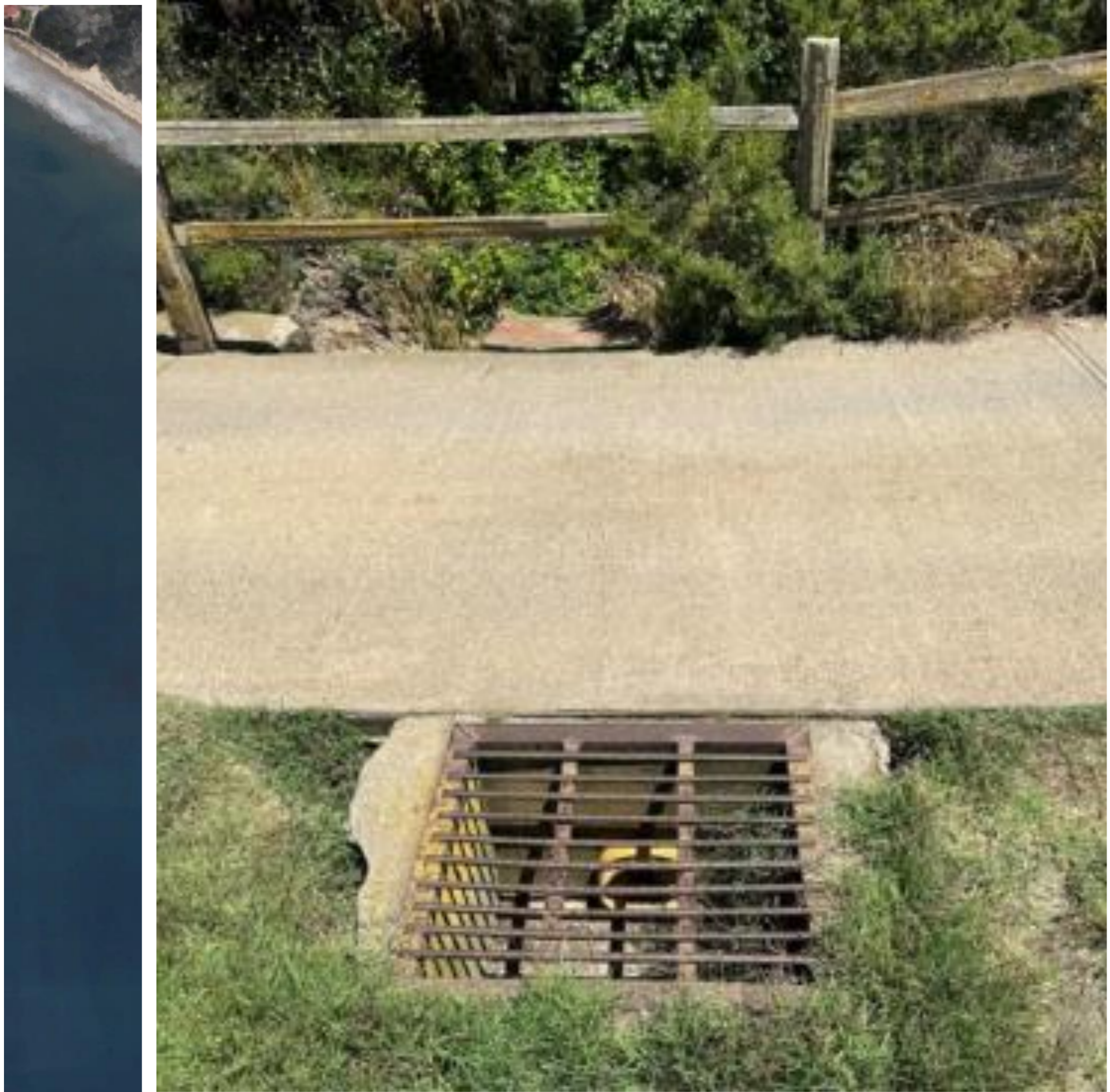
Current culvert by cart path
