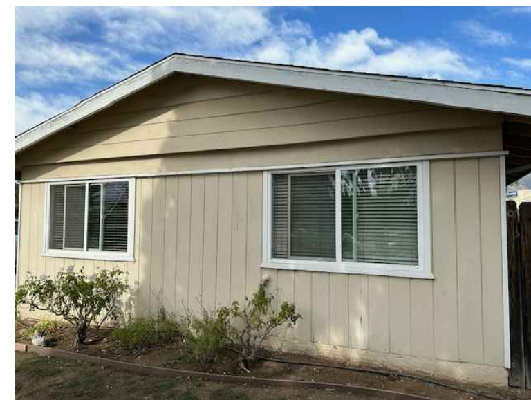
STREET VIEW - DEL NORTE DRIVE - SOUTH
