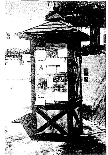
Figure 34 - Kiosk, Carpinteria, CA
