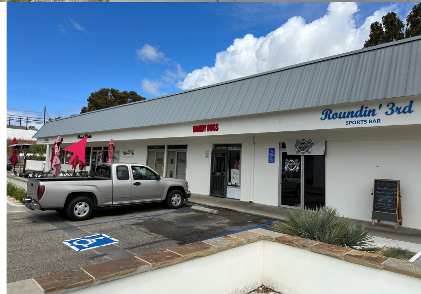
View of property from parking lot showing neighboring signs
