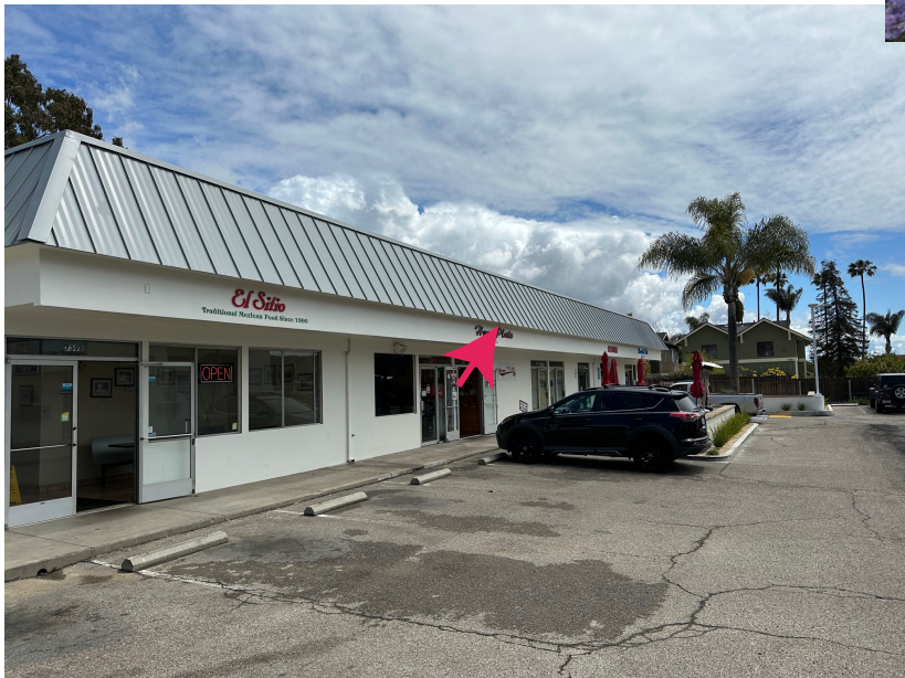
View of property from parking lot showing neighboring signs
