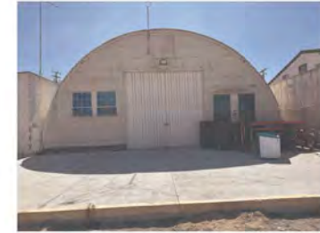
EXISTING QUONSET HUT #1
