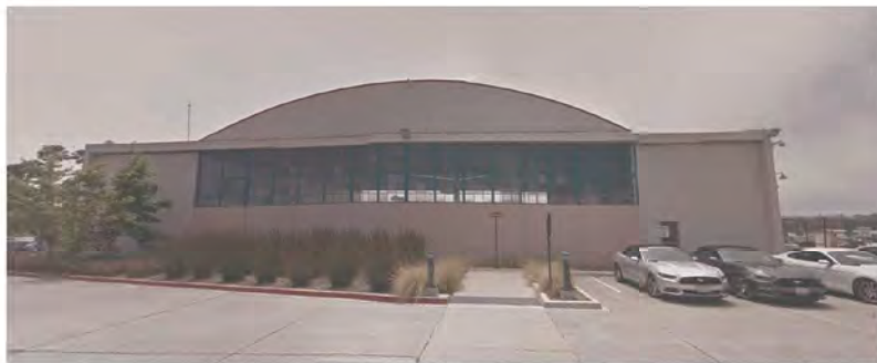
VIEW OF EXISTING HANGAR FROM AIRPORT EXIT
