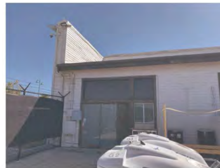
EXISTING HANGAR FENESTRATION
