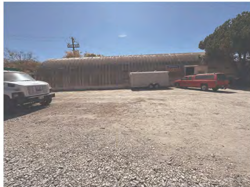
EXISTING QUONSET HUT #2
