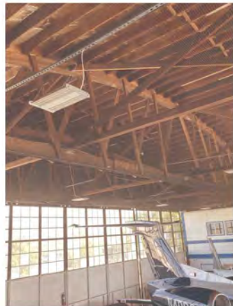
EXISTING TRUSSES & DOORS
