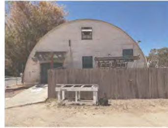
EXISTING QUONSET HUT #2
