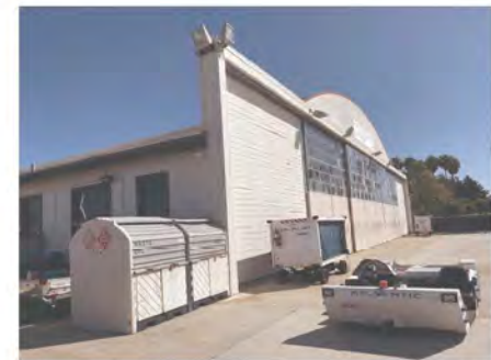
EXISTING HANGAR DOORS
