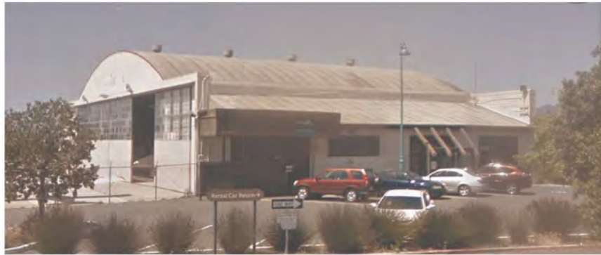
VIEW OF EXISTING HANGAR FROM MOFFETT PL
