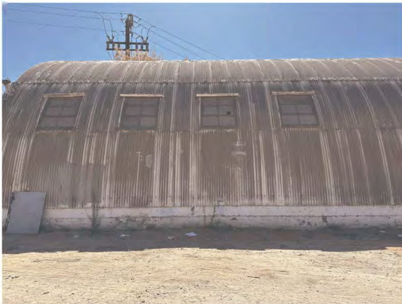
EXISTING QUONSET HUT #2
