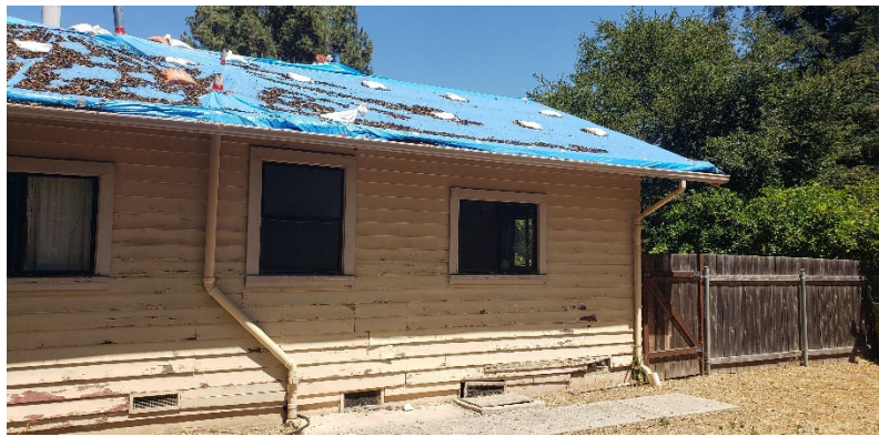
BACK OF FACILITY
