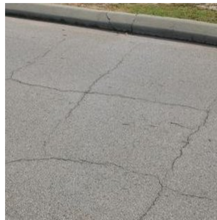
Block Cracking
