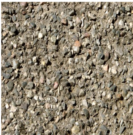
Weathering or Raveling
