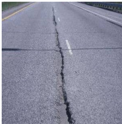
Transverse or Longitudinal Cracking
