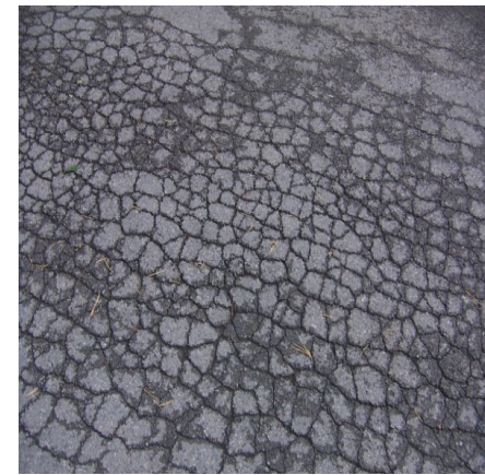
Alligator Cracking
