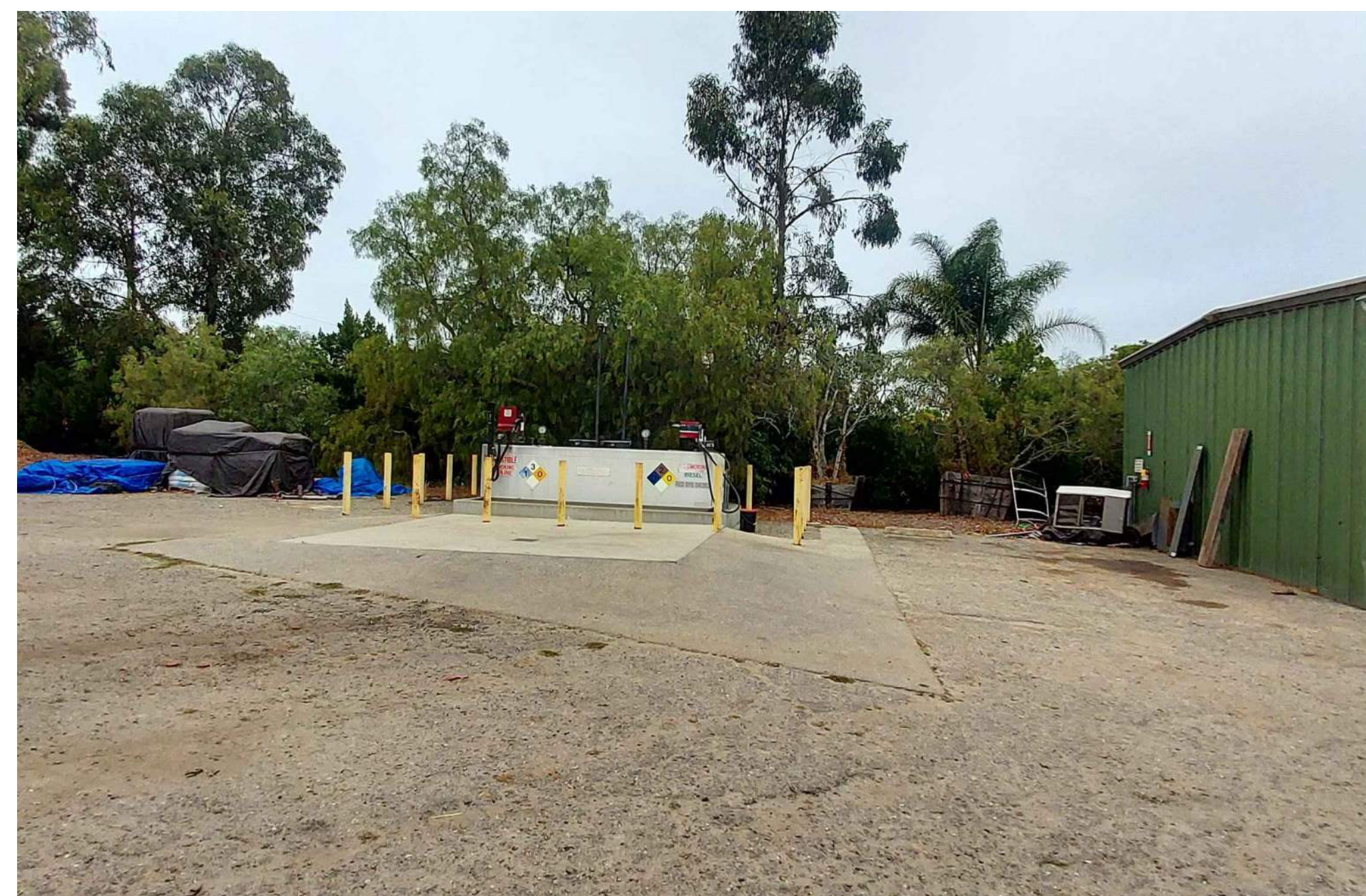
3 FUEL STATION EAST VIEW
