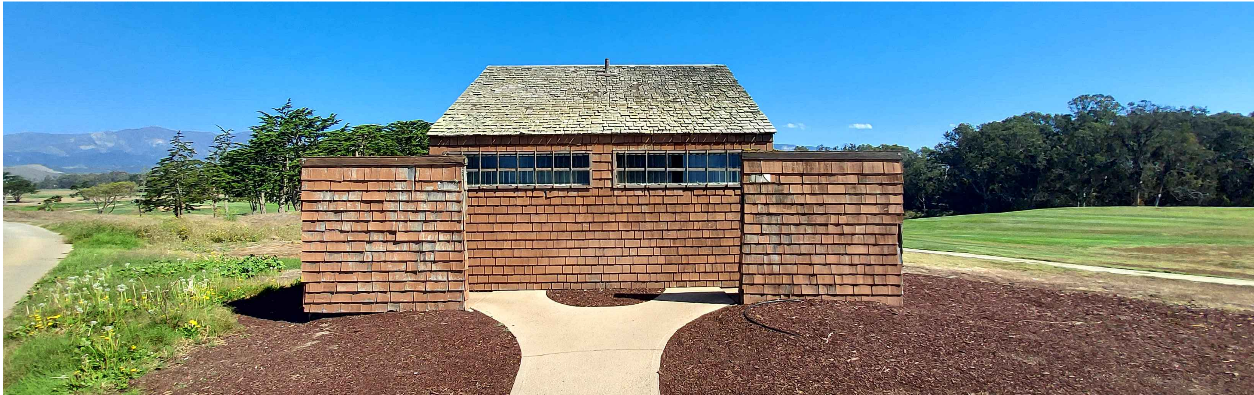
3 COMFORT STATION NORTH VIEW
