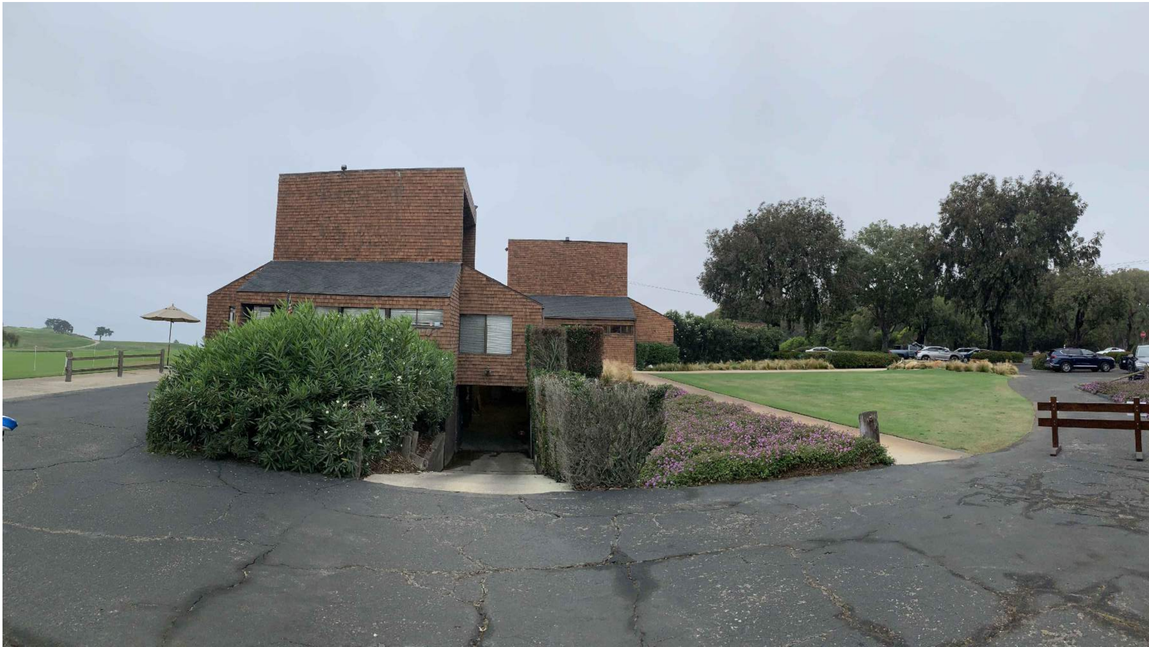
3 CLUB HOUSE BASEMENT EAST ENTRANCE
