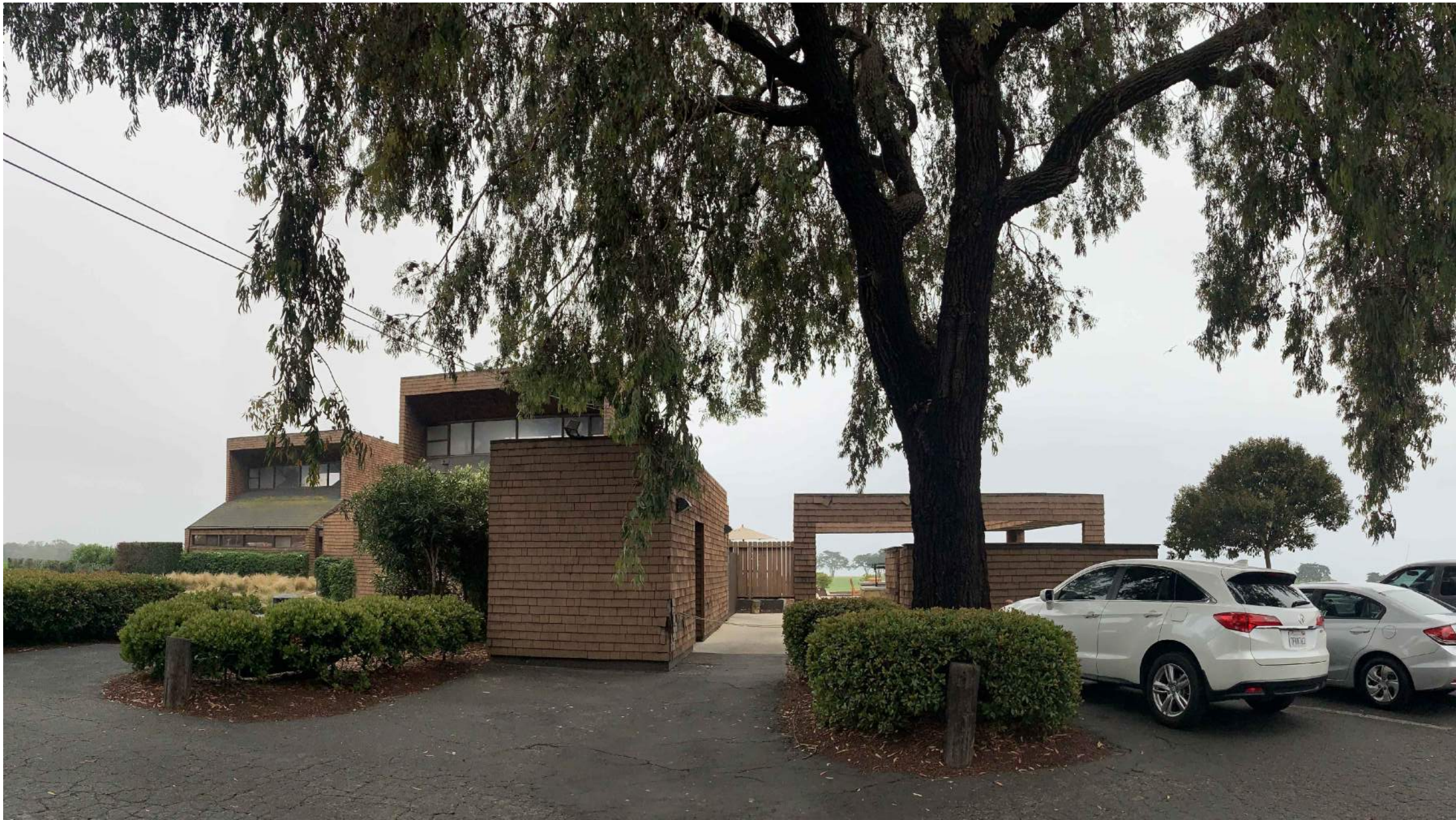
4 CLUB HOUSE SOUTH-EAST VIEW
