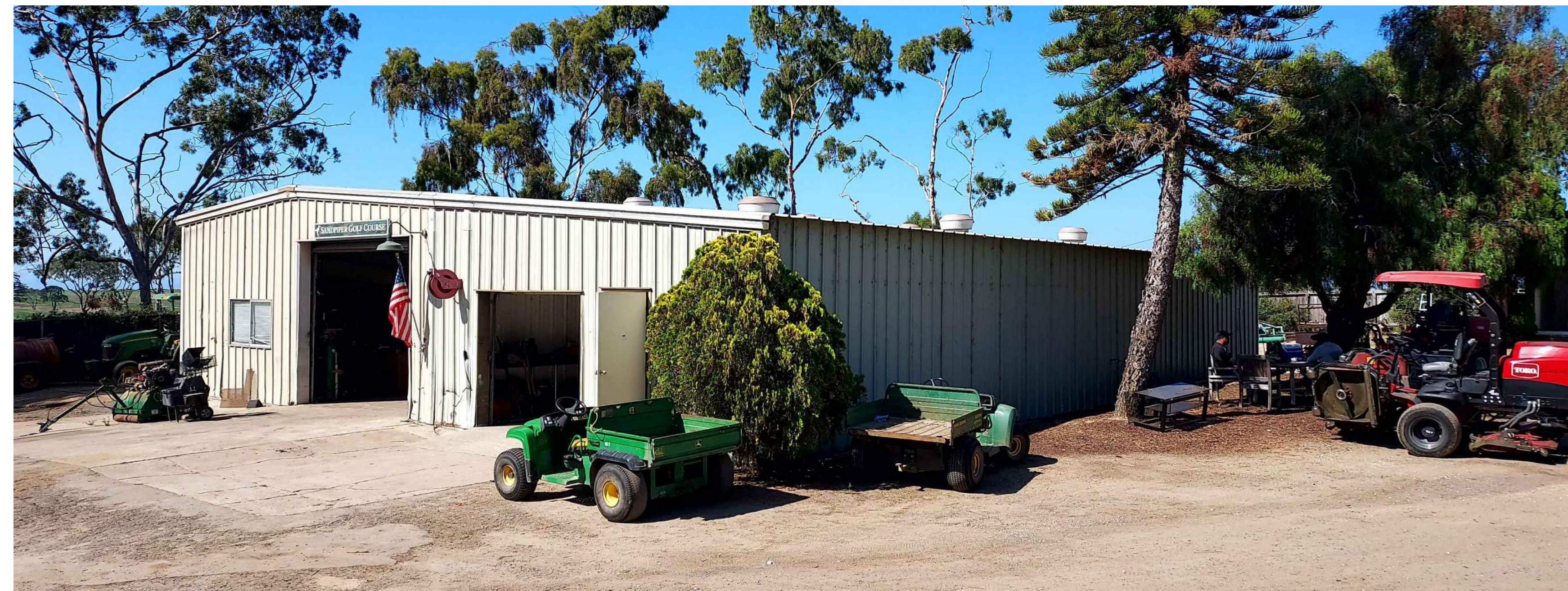
5 SMALL STORAGE / STAFF SOUTH-WEST VIEW
