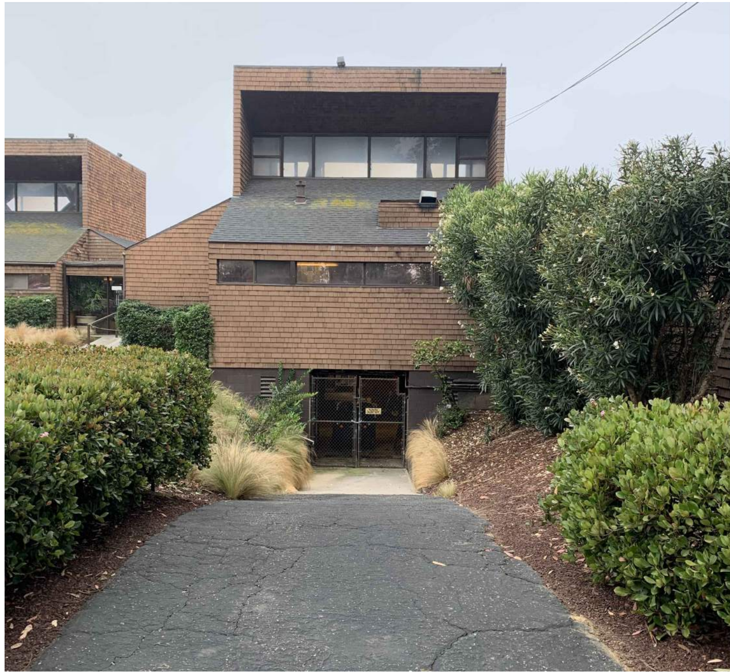
6 CLUB HOUSE BASEMENT NORTH ENTRANCE
