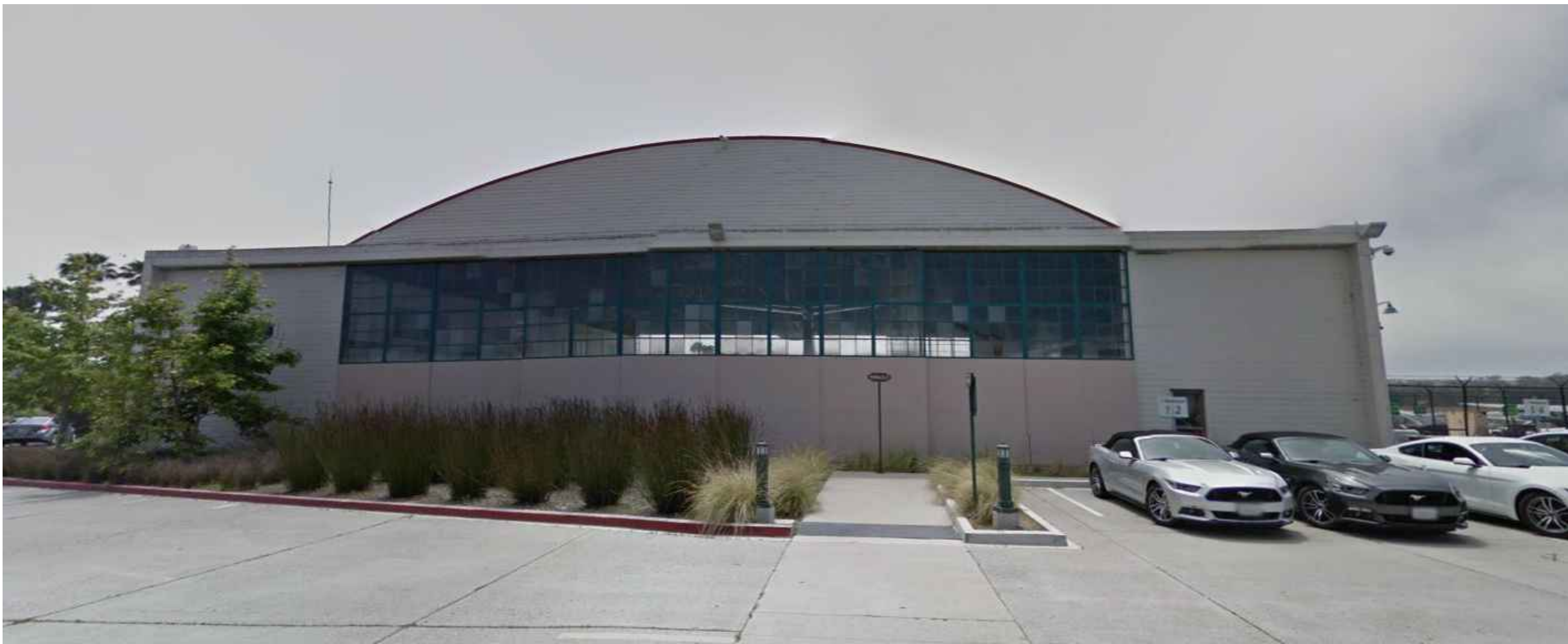
VIEW OF EXISTING HANGAR FROM AIRPORT EXIT
