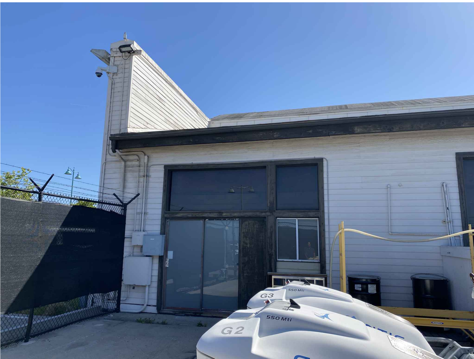
EXISTING HANGAR FENESTRATION
