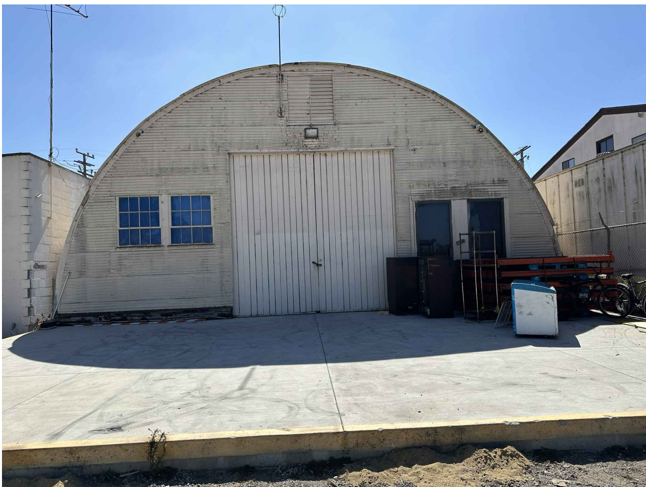
EXISTING QUONSET HUT #1
