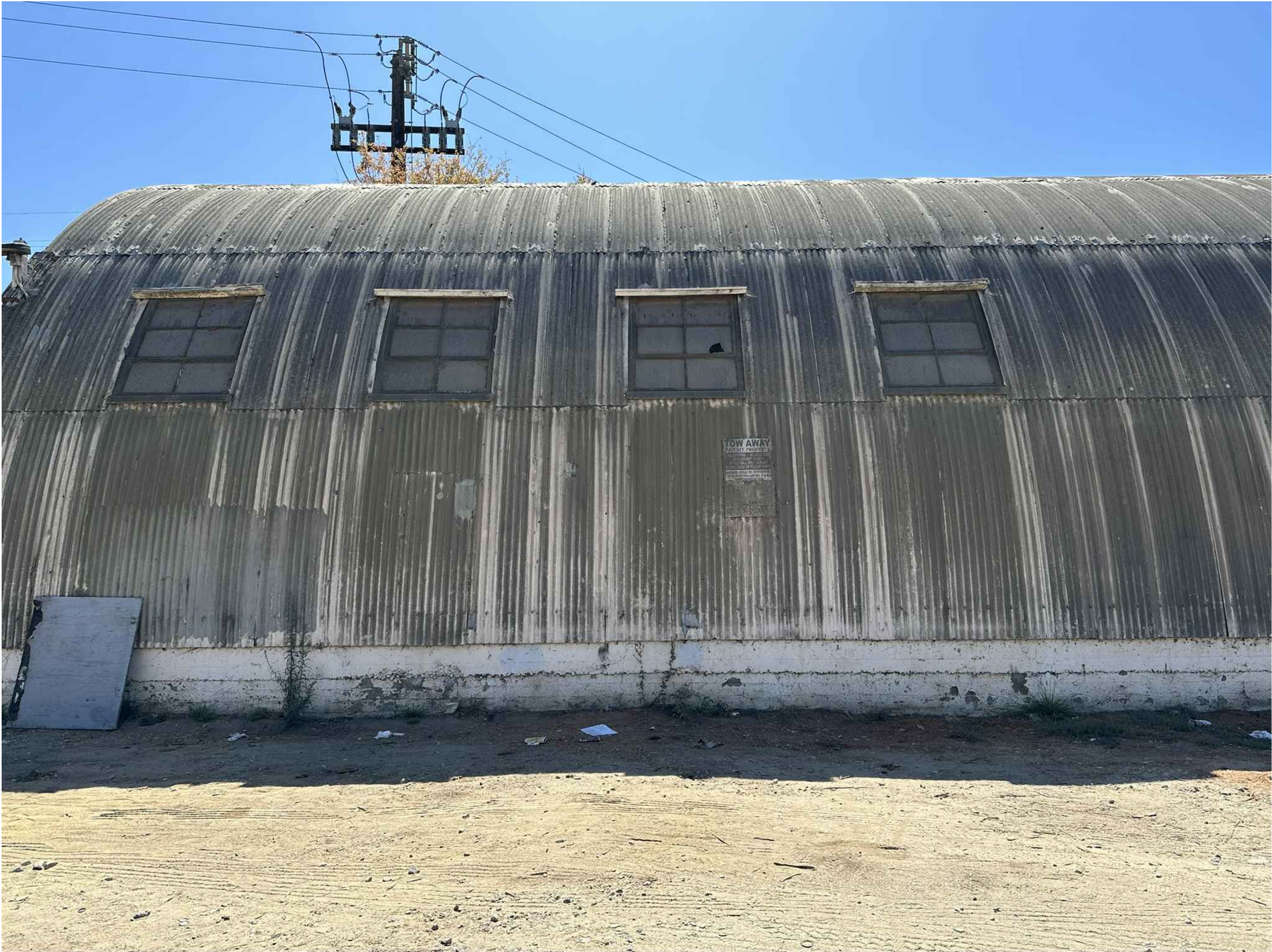
EXISTING QUONSET HUT #2
