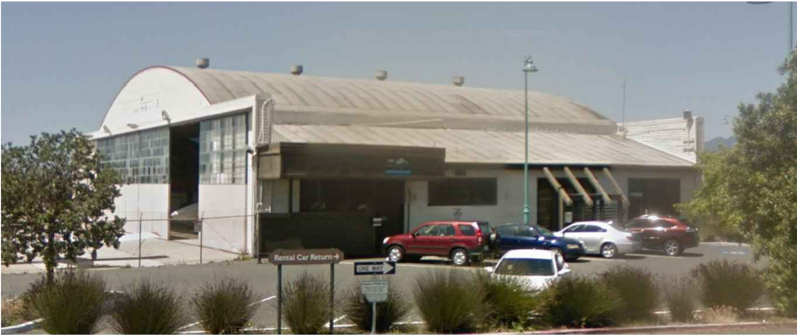
VIEW OF EXISTING HANGAR FROM MOFFETT PL
