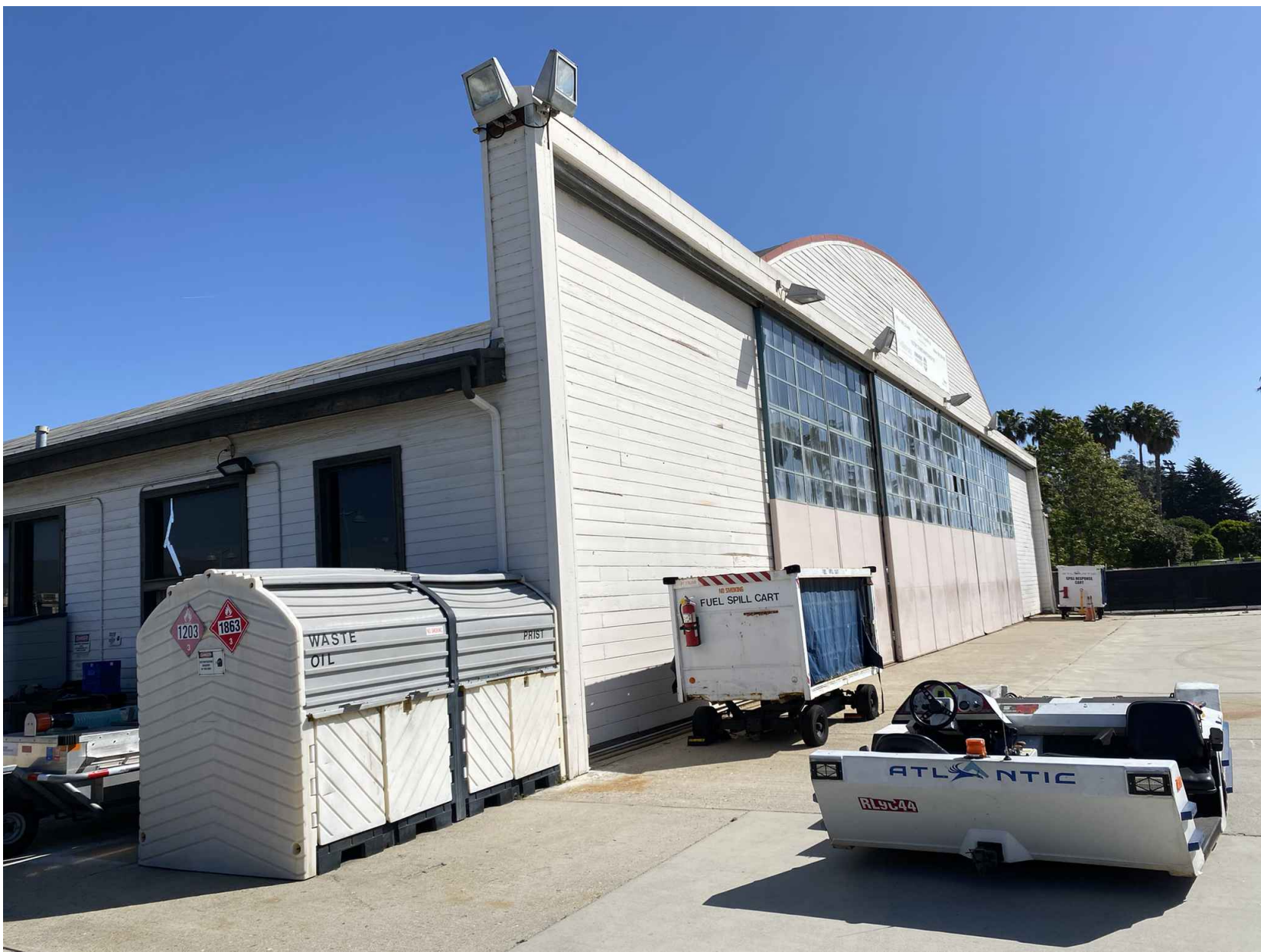
EXISTING HANGAR DOORS
