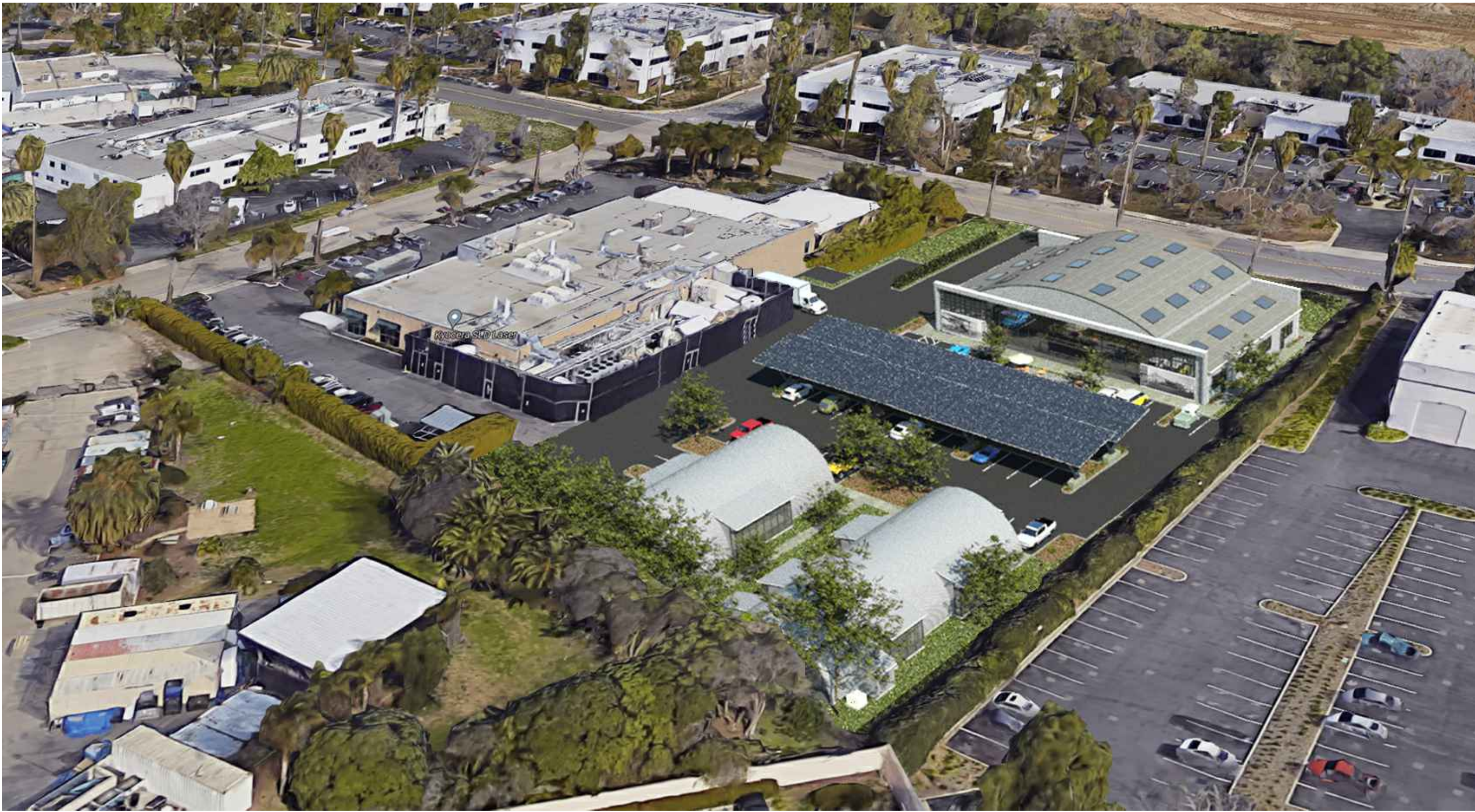
BIRD'S EYE VIEW OF SITE FROM SOUTH
