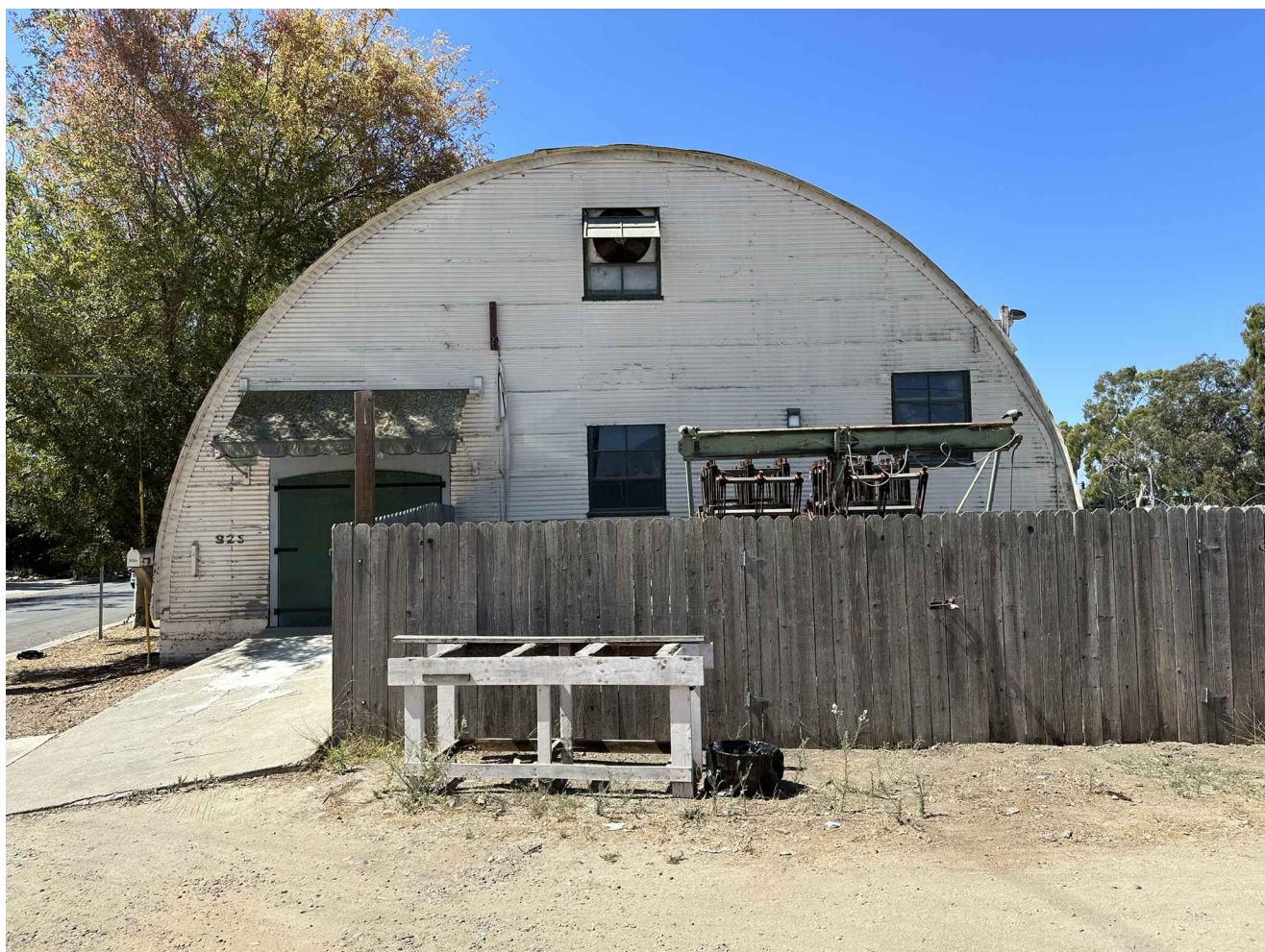
EXISTING QUONSET HUT #2
