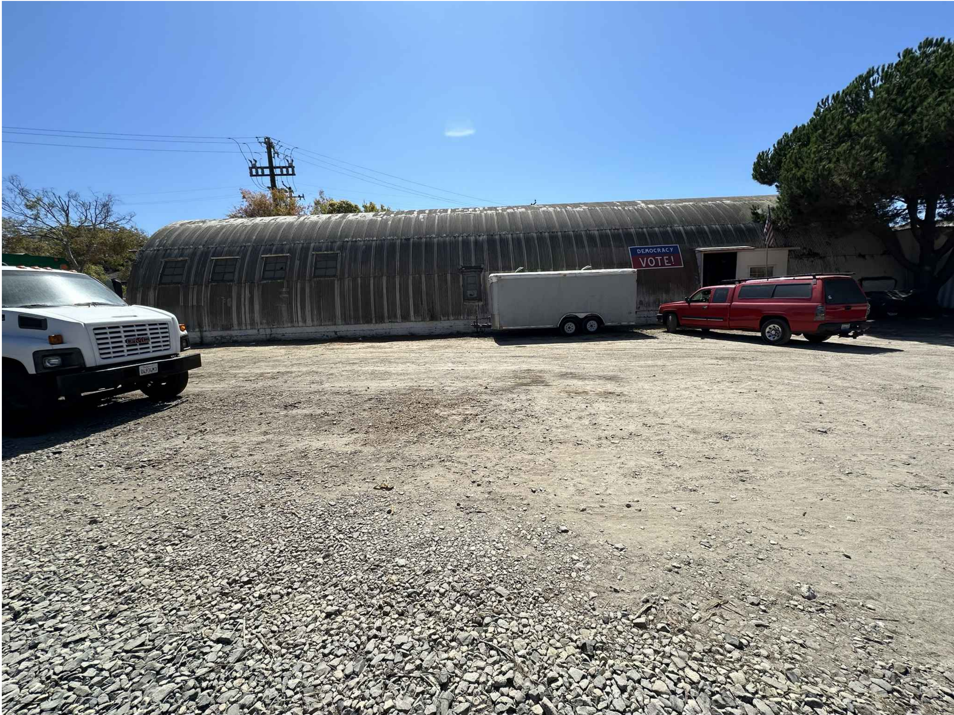
EXISTING QUONSET HUT #2
