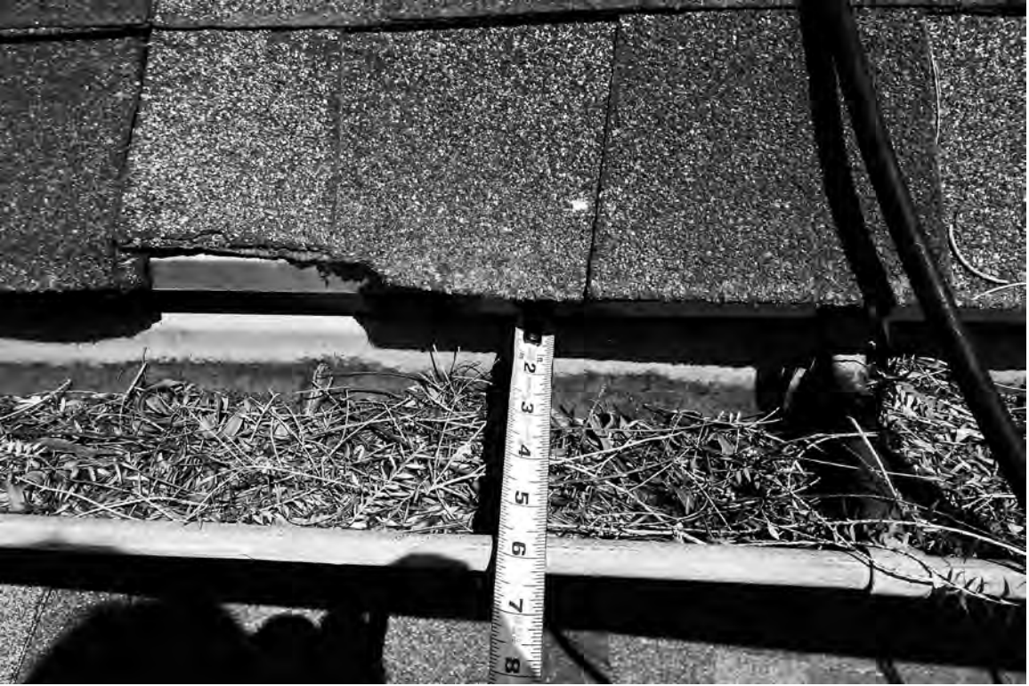
M. Typical Half-Round Gutter
