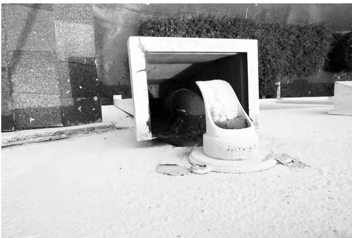
J. Typ. Conductor Head w/ Overflow
