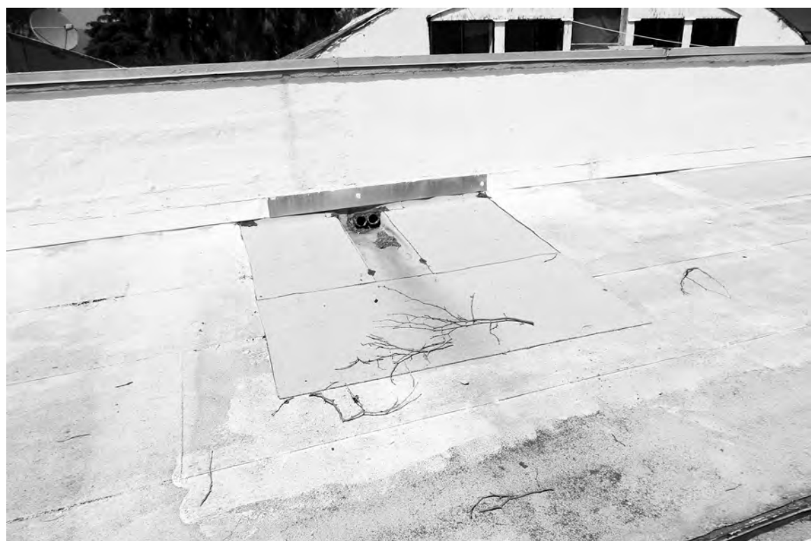
R. Through-Wall Drainage
