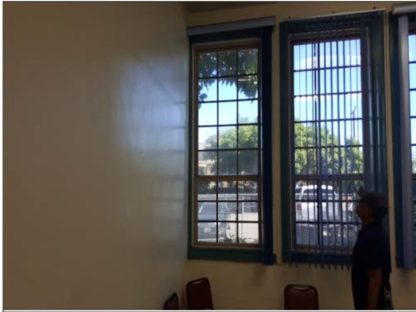
Residential-grade windows with failed jamb opening system at Community Center
