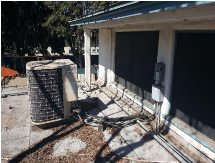
Condenser unit for Building B appear inoperative.
