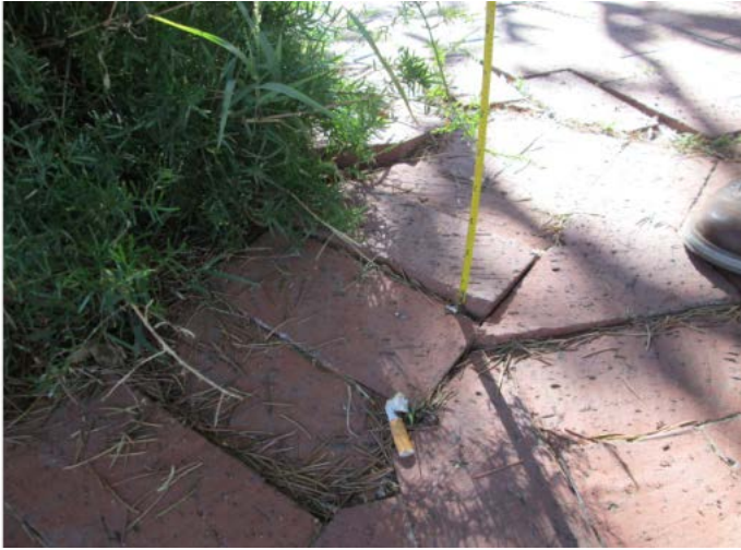
Uneven pavers at accessible route from Hollister Avenue .
