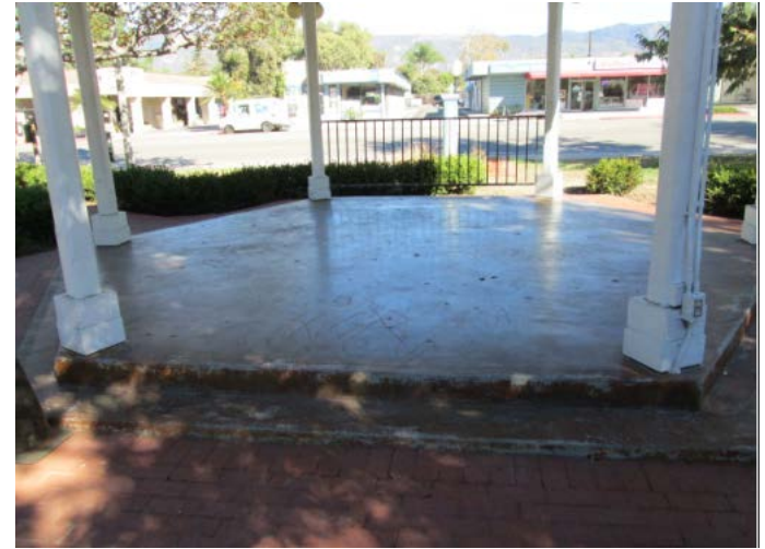
Accessible ramp required to top level of gazebo .
