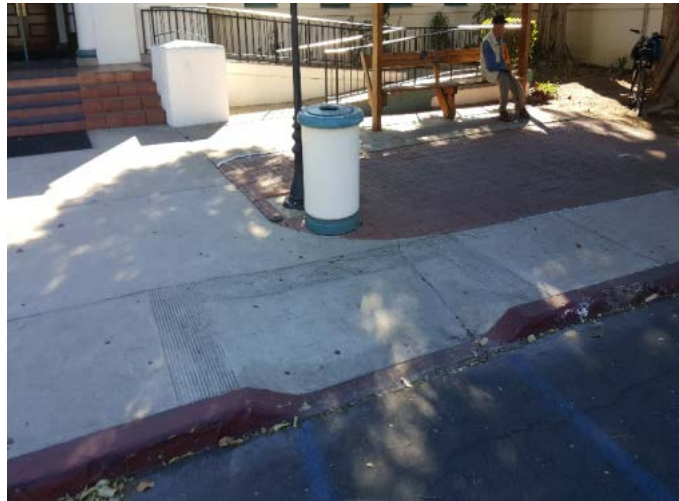
Non-compliant curb cut at sidewalk from accessible route.
