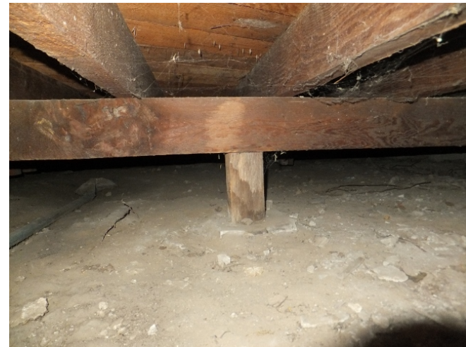
Main Building A substructure pier and floor framing.
