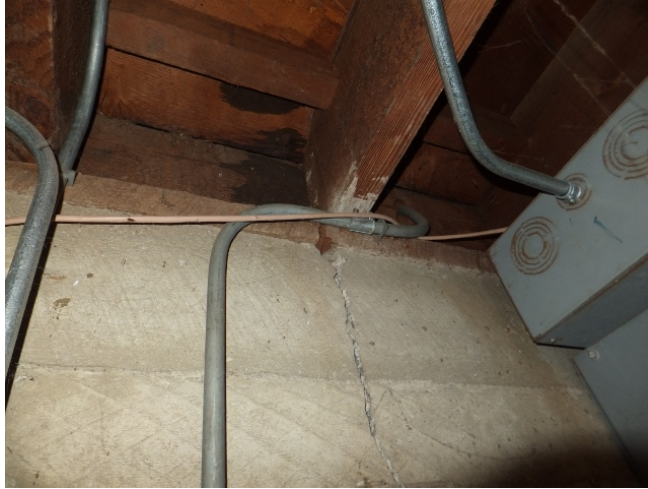
Basement wall foundation and sill plate with vertical split is widest at the top and narrower at the floor
