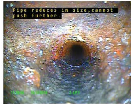
Line reduces in size unable to push further past 2.40 ft.
