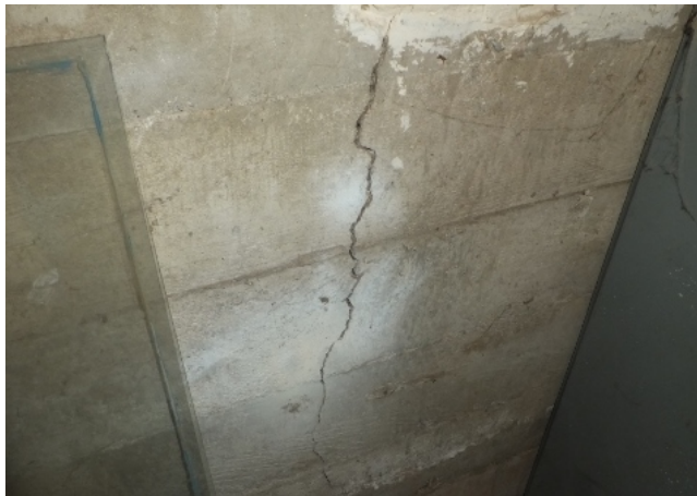
Vertical crack in basement foundation wall, Main Building A
