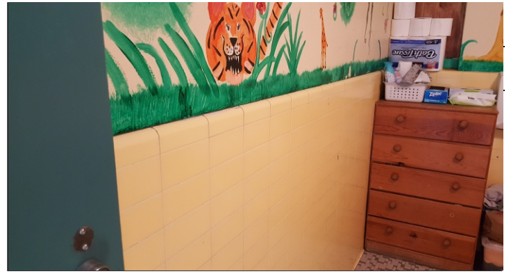
12. View of the lead containing ceramic tiles.
