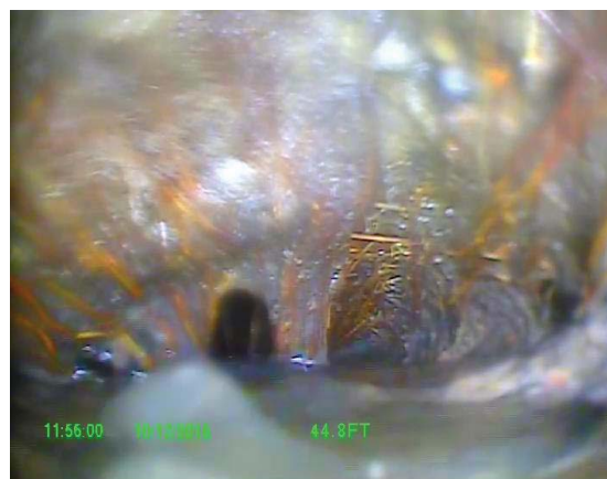
Debris at bottom of line at 38.30 ft.
