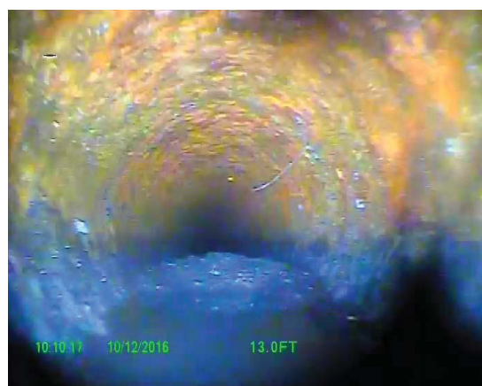
Debris at 13.00 at bottom of line.
