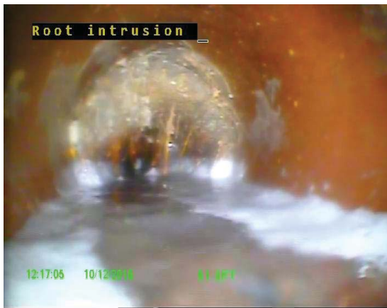
Unable to push past 50.40 ft. due to blockage with debris. Heavy root intrusion at 51.30 ft.
