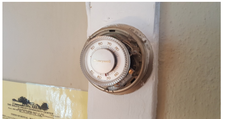
8. View of the mercury thermostats.
