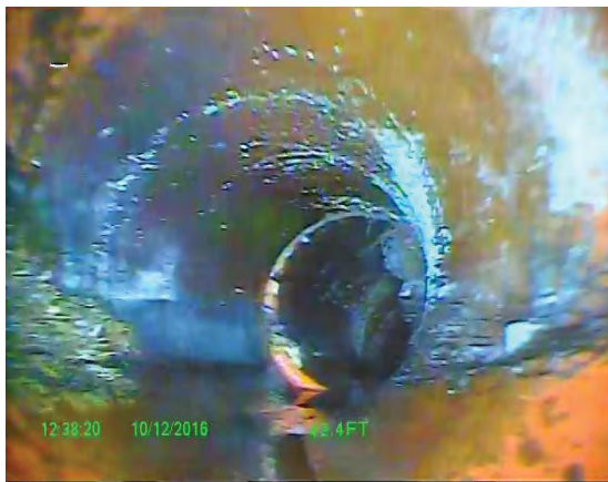
Line turns right at 42.40 ft. with root intrusion.
