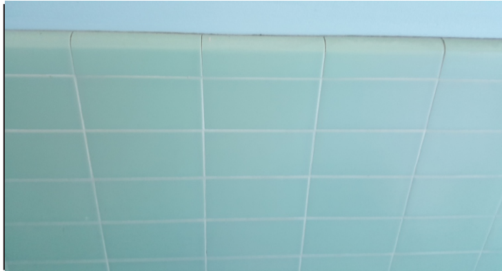
11. View of the lead containing ceramic tiles.
