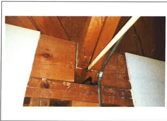
27. Barrel truss tie rod bottom chord and bearing top plate of short wall above original concrete walls of Assembly Room
