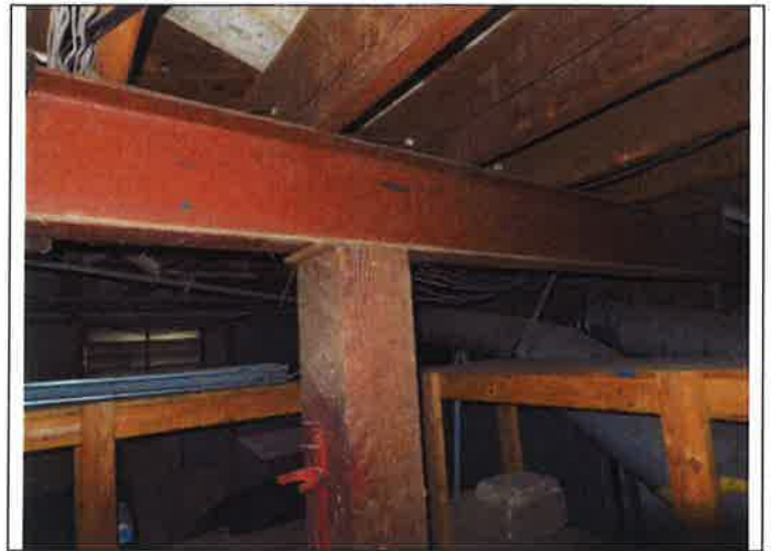
14. Basement floor joists, steel girder and wood post
