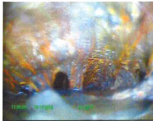
Debris at bottom of line at 38.30 ft.
