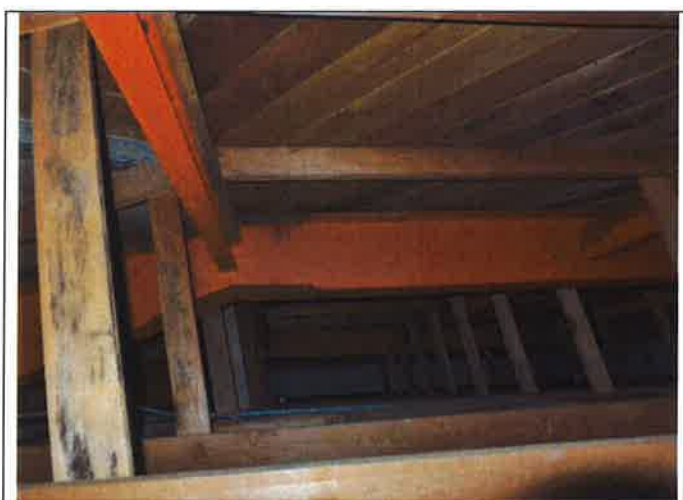
58. Steel and wood framed roof over Classroom Building B
