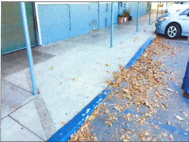
9. Non-compliant ADA curb cut along Building C4
