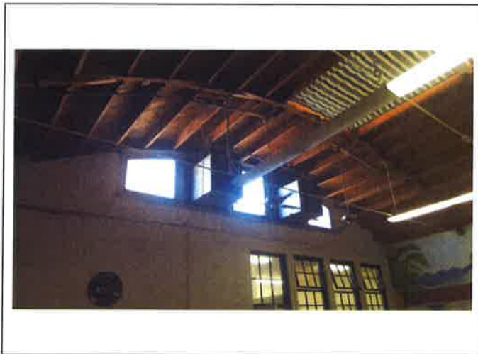
25. Barrel truss roof over Assembly Room and short framed wall looking north over kitchen windows, Main Building A
