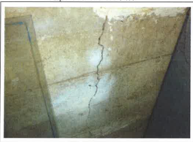
11. Vertical crack in basement foundation wall, Main Building A
