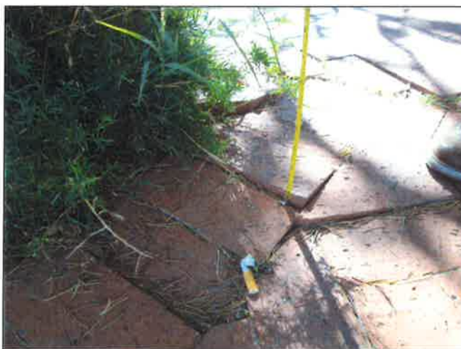
29. Uneven pavers at accessible route from Hollister Avenue
