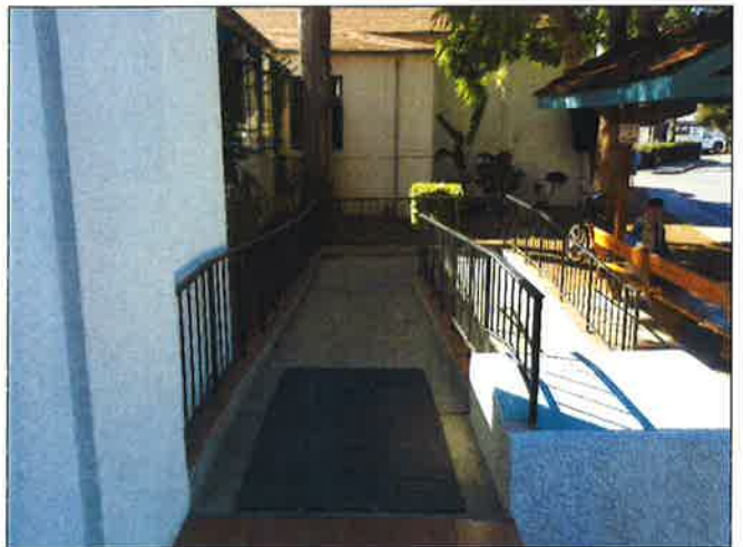
102. Non-compliant handrails at ADA ramp to main entrance
