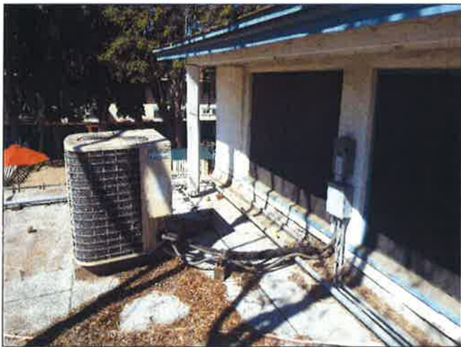
99. Condenser unit for Building B appears inoperative
