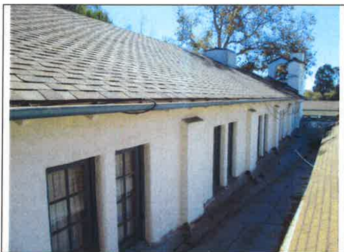
33. Upper windows of Auditorium, cricket over sloped roof of original hallway and Assembly Room roof on right
