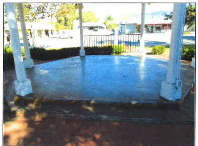
30. Accessible ramp required to top level of gazebo
