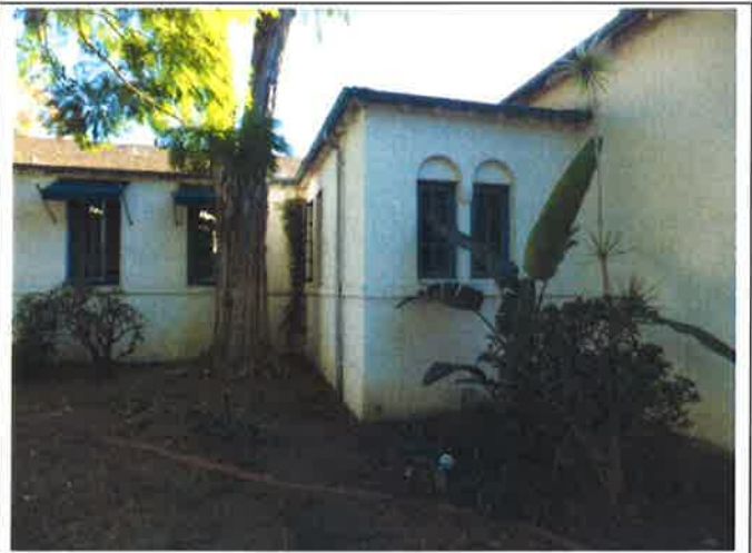
5. Main Building A, Spanish style architecture is missing the original red clay tile roof, replaced by composition shingles
