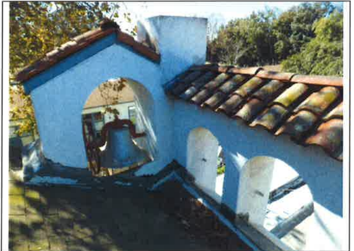
6. Red clay tile roof on a bit of wall at southwest corner of Auditorium shows original roof covering.
