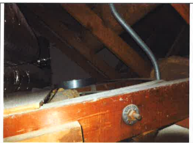
57. Wood framed truss roof over Classroom Building C4
