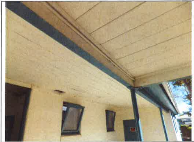
43. Fixed, rigid connection of walkway roof at Main Building A
