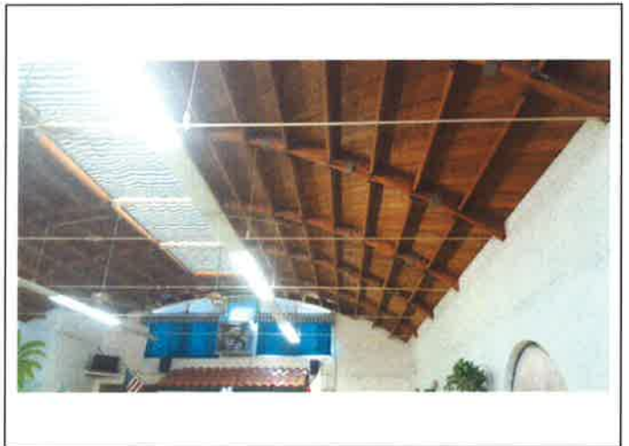
24. Barrel truss roof over Assembly Room looking south over stage, Main Building A
