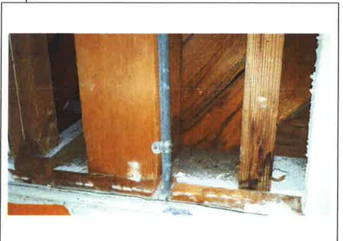
30. Posts and studs of short cripple wall above original concrete wall over Assembly Room, Main Building A
