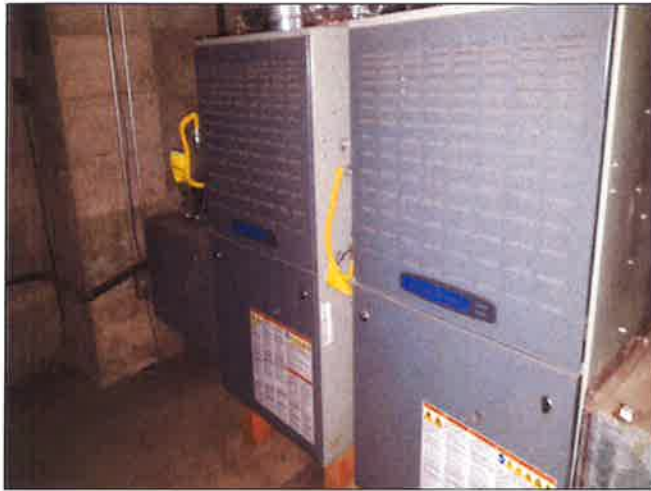
97. Furnaces for Community Center classroom's heaters at basement
