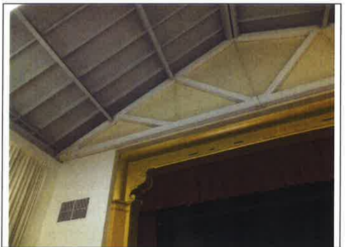
16. Auditorium Roof truss over stage opening
