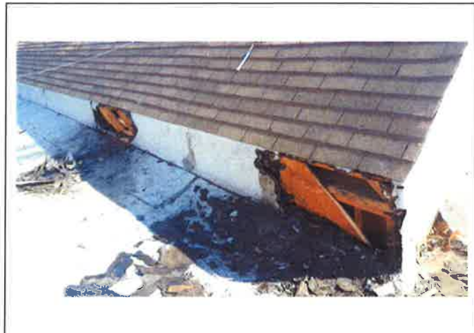
32. Diagonal wall sheathing of short wall at Assembly Room roof
