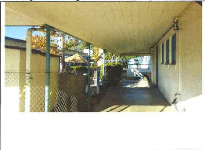
47. Covered walkway roof with fixed connections to Main Building A at south wall at east wing on right
