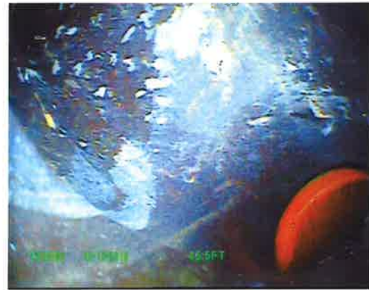
Line drops at 45.50 ft with lateral on left.
