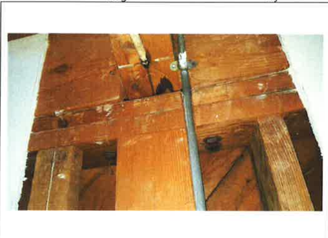
29. Barrel truss bearing plate anchor bolts in top plate, post and studs below truss in short wall above original concrete wall
