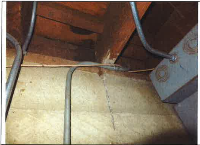
9. Basement wall foundation and sill plate with vertical split is widest at the top and narrower at the floor
