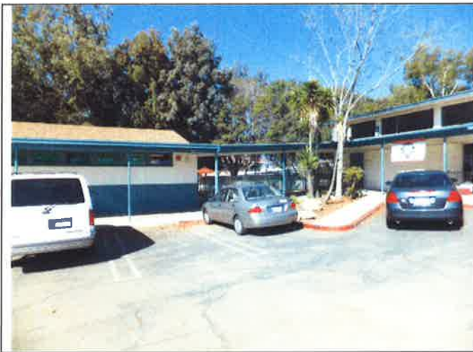
45. Covered walkway roof with fixed connections to Building B on right and Building C4 on left
