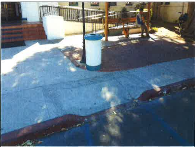
101. Non-compliant curb cut at sidewalk from accessible route
