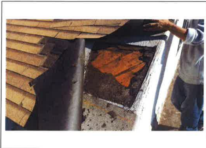
31. Roof covering removed over diagonal sheathing at south end of Assembly Room roof, Main Building A
