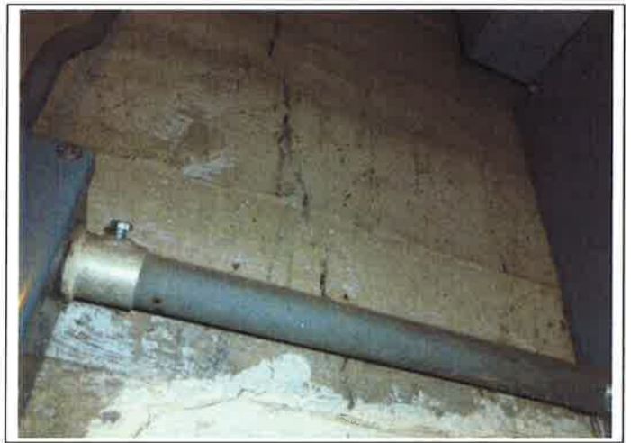
10. Vertical crack in basement foundation wall, Main Building A
