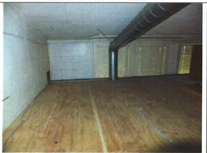
59. Loft floor and original ceiling above offices in Classroom Building B, High windows beyond, new ceiling below
