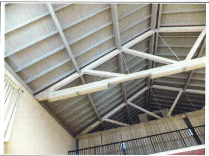
15. Auditorium roof trusses, purlins, rafters and T&G sheathing, Main Building A
