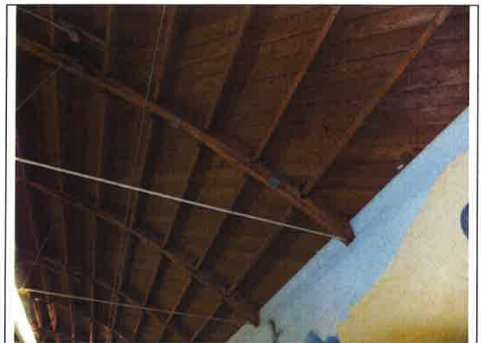
26. Barrel trusses, 2x rafters and diagonal sheathing over Assembly Room, white tie rods as bottom chords
