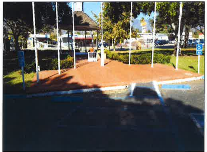
100. Curb ramps are non-compliant and requires reconfiguration
