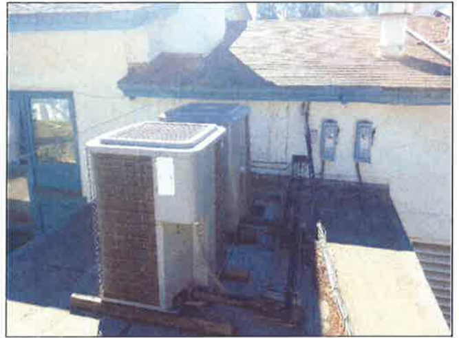
98. Condenser units at roof
