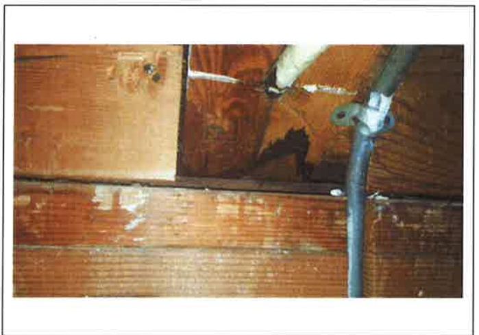
28. Barrel truss bearing plate and tie rod end plate, after wall plaster was removed
