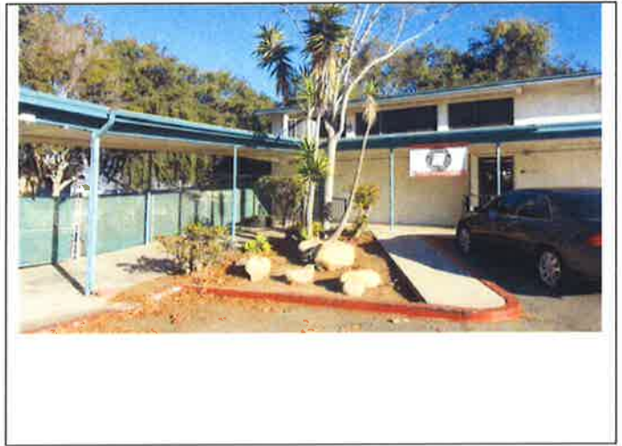
46. Covered walkway roof, fixed connections to Building B on right and Building C4 on left
