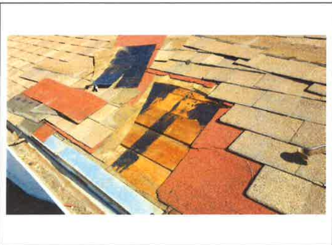
23. Auditorium roof with roof covering peeled back to expose 1x sheathing
