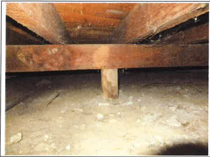
7. Main Building A substructure pier and floor framing
