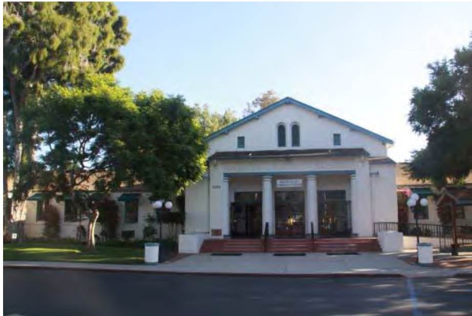
Figure 2 - Front Entrance of Building A
