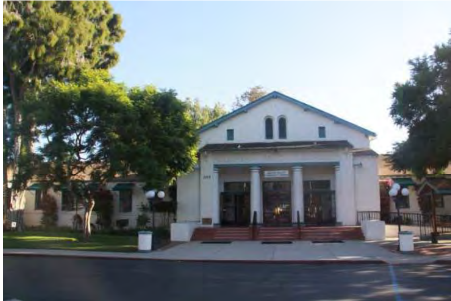
Figure 1 - Front Entrance of Building A
