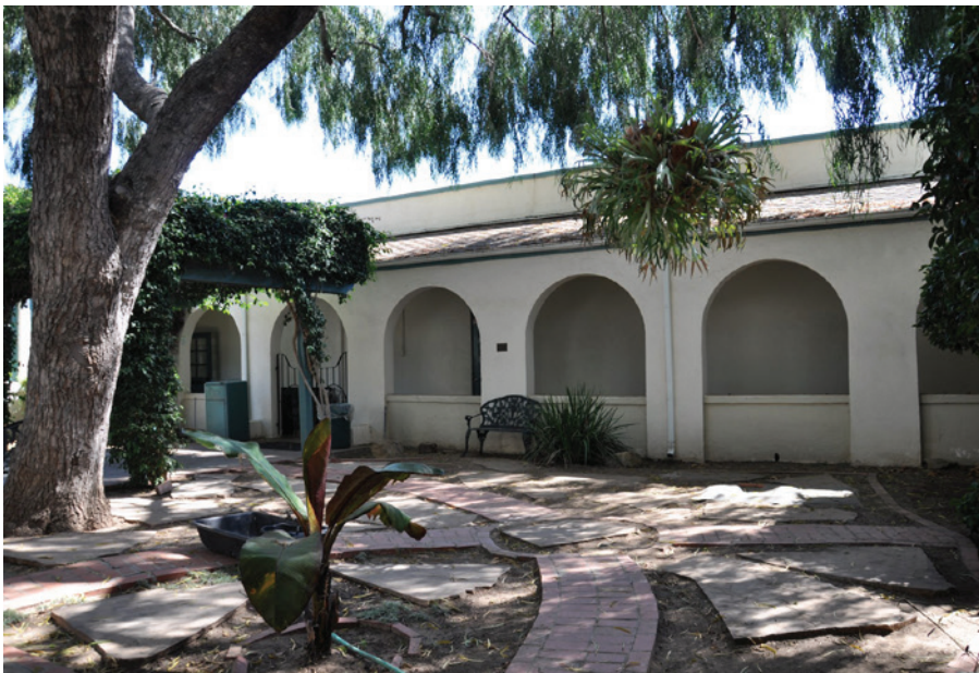
Figure 7. East patio, looking east at arched corridor.
