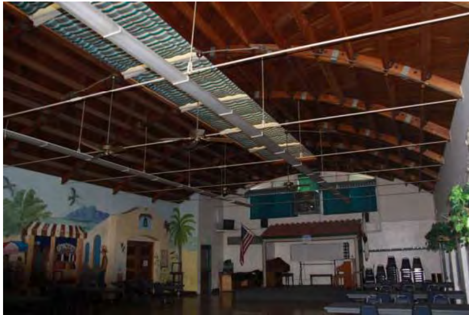
Figure 4 – Building A, Barrel Vaulted Roof Addition
