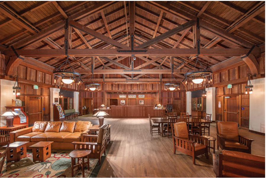
Figure 21. Sensitive installation of fire sprinkler and seismic reinforcement in architecturally significant interior spaces.
