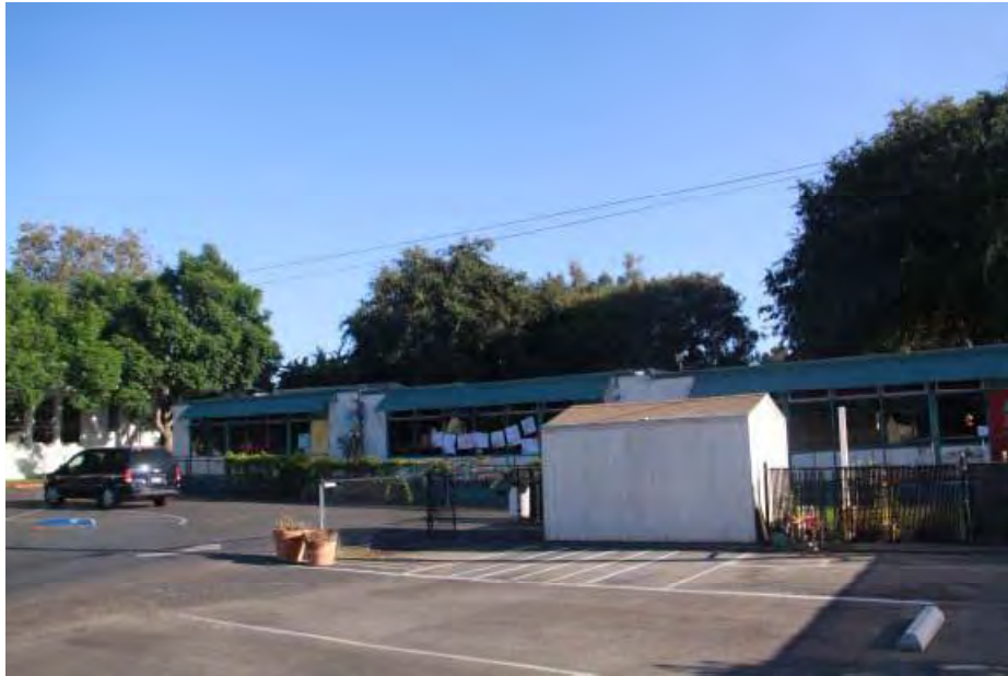
Figure 3 – Front of Building C2
