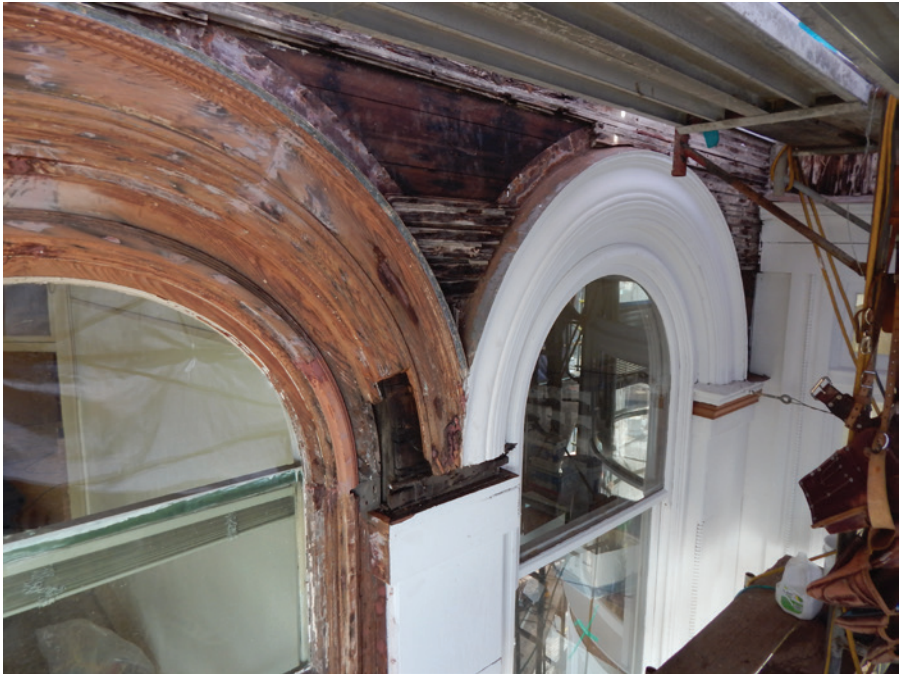
Figure 20. Wood repair and maintenance.
