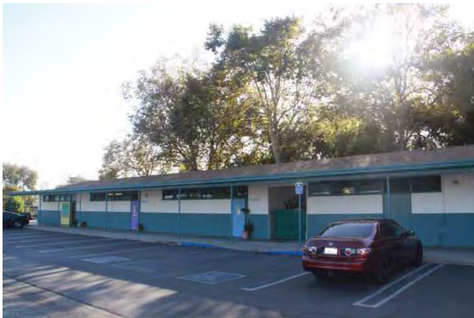
Figure 4 – Front of Building C4
