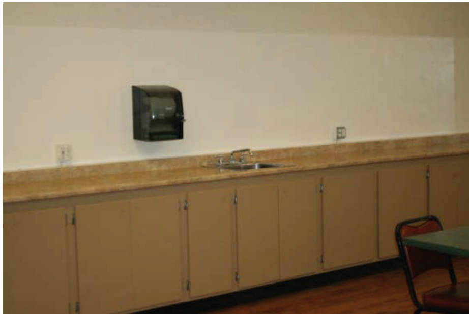
Figure 8 – Building A, non-compliant cabinet and sink
